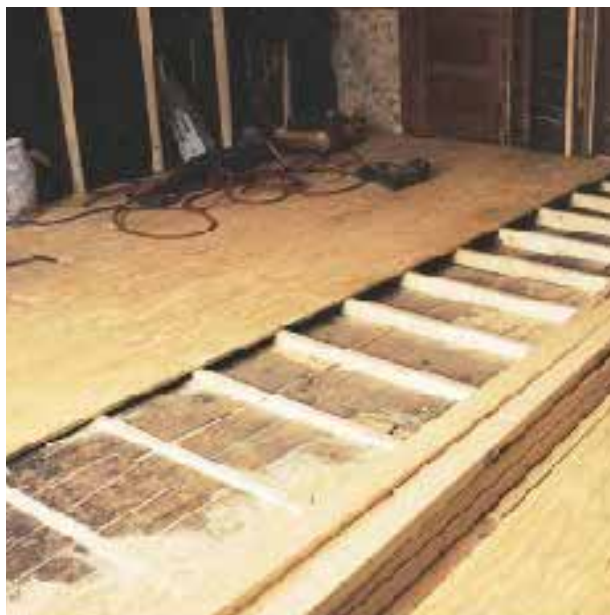
Figure 5. A new \frac{3}{4} -inch tongue-and-groove plywood subfloor provided a sound base for carpet and built-ins.
