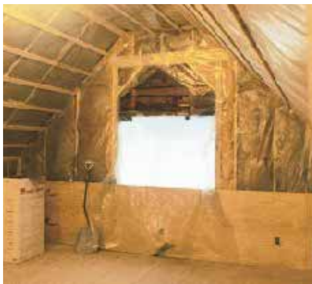
Figure 6. Prepped for finishes, the new attic room has straight ceiling lines, a level floor, and a much stronger roof. Along the bottom of the walls, plywood provides solid nailing for paneled wainscoting.
