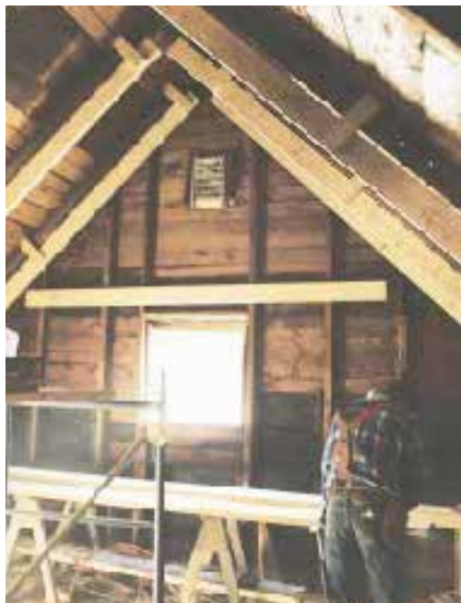
Figure 1. New 2x6s sistered onto the undersized existing rafters matched the drywall plane formed by new 2x12 rafters.
