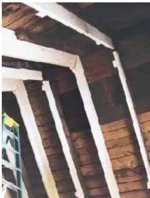
Figure 2. New 2x12 rafters were installed between existing rafters to strengthen the roof framing. There was enough give to the old roof sheathing so that the new rafters could be installed without having to fiddle with jacks — a sledgehammer did the job.
