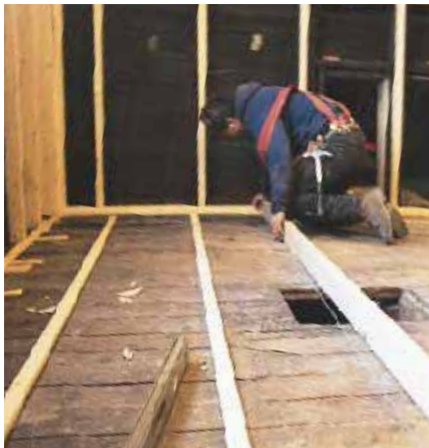
Figure 4. After installing a level nailing strip around the perimeter of the room, the author snapped cut lines on each sleeper. This scribed sleeper system leveled and took the sags out of the floor.
