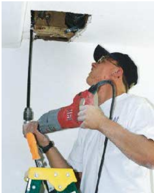
Figure 5. A heavy-duty right-angle drill is a necessity for boring joists and studs.
