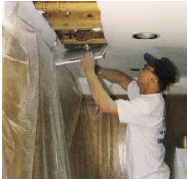
Figure 4. Marking precise cuts in drywall and saving the cutouts for reuse later help keep the cost of a job down.
