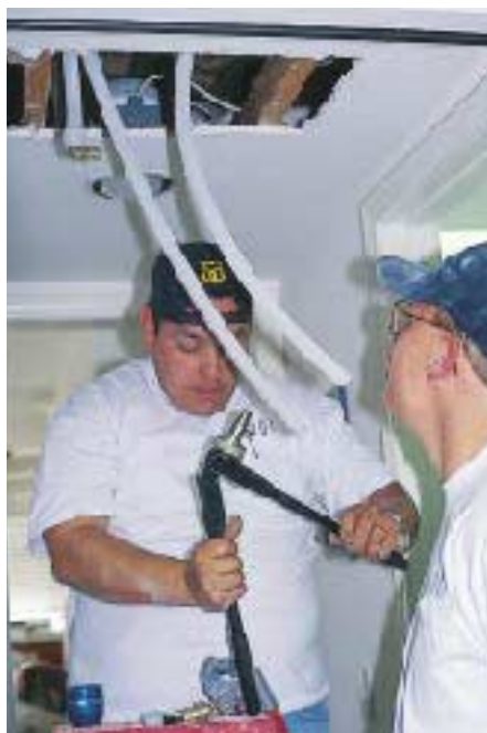
Figure 7. Wirsbo's PEX connects to brass fittings using a proprietary expansion tool bit (left). The cut end of the PEX is expanded, the fitting slides into place (right), and within seconds, the PEX contracts back to its original diameter. Rings placed outside the cut end ensure strong, leak-free connections.
