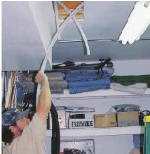
Figure 6. Hot and cold PEX water lines are strapped together for feeding into cutouts.
