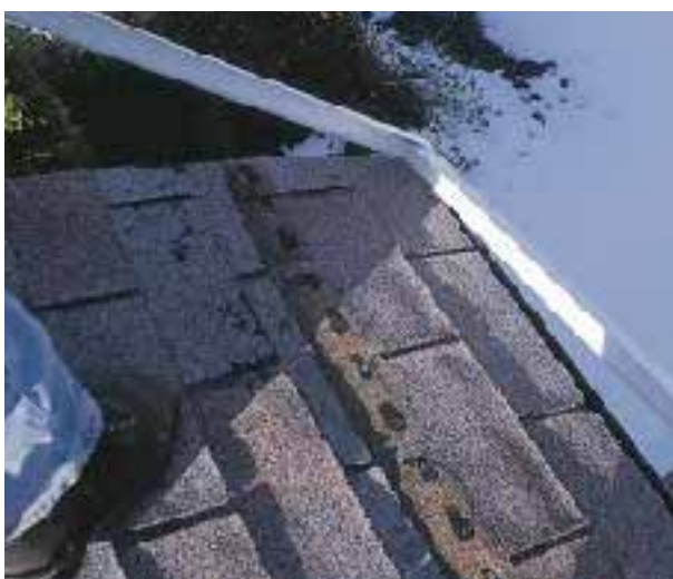
Figure 2. Depending on the type of job, the author uses several specialty drip edge profiles, including one with an extra-long leg designed to cover existing shingles and drip edge (at right in photo above). A single length of drip edge wraps roof corners, with the rake flashing overlapping the eaves for good drainage (right).
