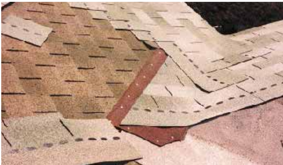
Figure 6. Valleys are first flashed with 90-pound roll roofing. Then shingles from one roof plane are laid so they extend one tab beyond the valley center. Shingles from the other roof plane are overlaid, then cut back with a hooked knife to form a “closed” valley.
