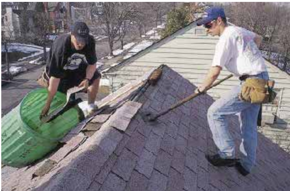
Figure 1. The roofing crew uses a Red Ripper roofing demolition tool to pry up cap shingles, which are collected in a plastic bin, along with old boot flanges and any loose shingle tabs.
