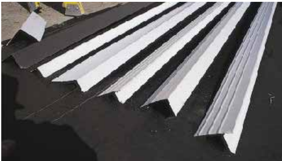
Figure 2. Depending on the type of job, the author uses several specialty drip edge profiles, including one with an extra-long leg designed to cover existing shingles and drip edge (at right in photo above). A single length of drip edge wraps roof corners, with the rake flashing overlapping the eaves for good drainage (right).
