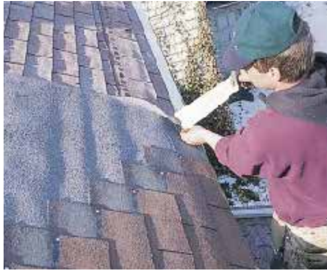
Figure 3. To guard against damage from ice dams, a 36-inch-wide strip of bituminous membrane is rolled out along the eaves. After lightly nailing the top edge, the membrane’s 4-inch-wide adhesive strip is pressed onto the new drip edge to form a tight seal.
