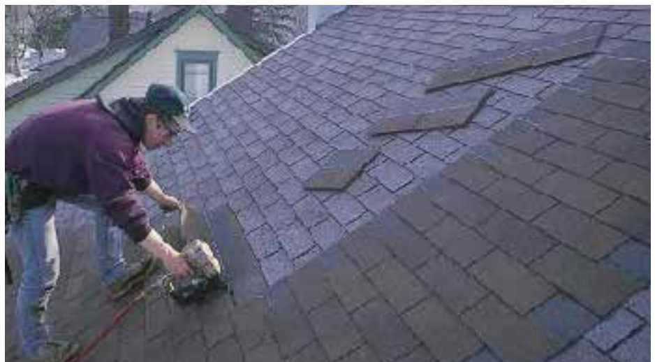
Figure 5. Every six courses, roofers on either side of the center column of shingles fill in a triangular area using pairs of three-, two-, and one-tab shingles (illustration). This resulting “pyramid” pattern ensures proper alignment of the tabs and enables several roofers to work without getting in one another’s way.
