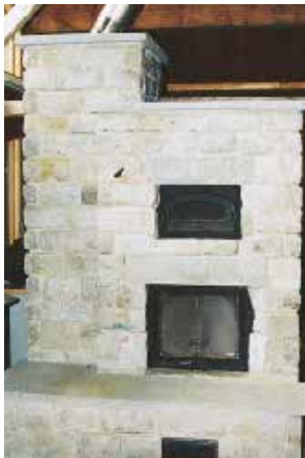
Figure 6. Masonry heaters, with their enormous thermal mass, are designed to burn very hot, then store and slowly release heat. Although more expensive than prefabricated metal fireplaces, they provide a reliable high-performance wood-burning hearth.
