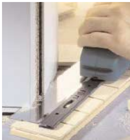
Figure 1. The Finecut Power Handsaw's flush-cutting blade makes it easy to trim door jambs and casing to allow room for flooring.
