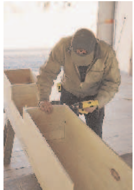
Figure 4. Four webs establish the width of the base.
