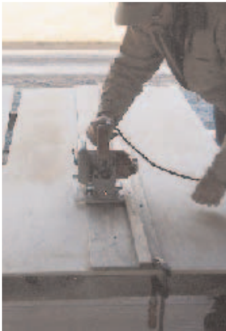
Figure 2. Both factory edges are used to provide a true plane for the top.
