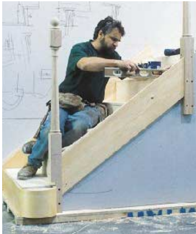
Figure 6: To scribe the face skirt, the author uses a level to mark true plumb and level cuts for each sub-riser and sub-tread.
