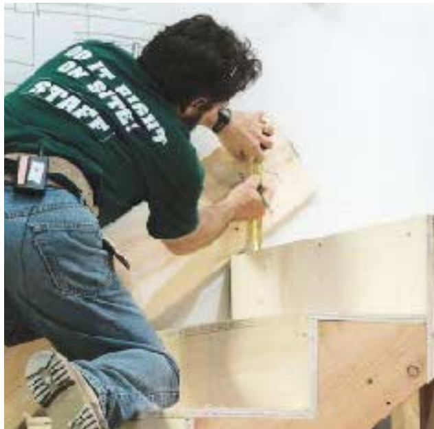
Figure 4: To notch the wall skirt around the landing framing, the author tacks the wall skirt along the nosings of the rough treads and marks a level line one standard rise above the landing floor.
