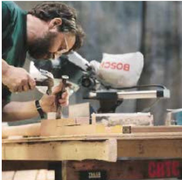
Figure 3: The author completes the newel pocket notches with a sharp chisel.
