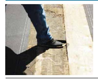
Problem: No support at sheathing edges. The plywood sheathing on this flat roof was installed without blocking under the edges. If someone walks on the roof, the roofing may crack when the sheathing flexes at the plywood joints.
