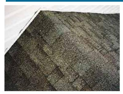
**Problem:** Exposed roofing nails. Exposed roofing nails are sometimes a source of leaks.
