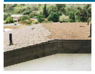
Problem: Because no gravel stop was installed, the asphalt flood coat and the roofing gravel are migrating down the face of the shingle roof.
