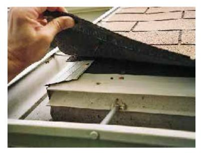
**Problem:** Valley shingles were not tabbed or spotted with roofing cement. The large volume of water that collects in a valley can back up under uncemented shingles.
