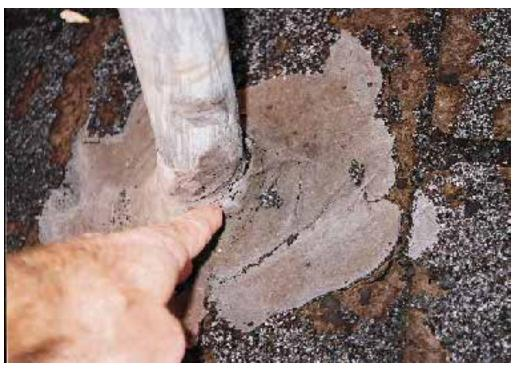
Careful flashing at penetrations and edges can prevent most roof leaks
