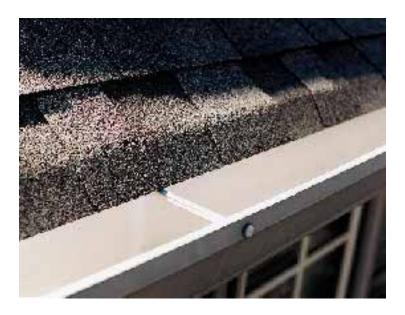
Problem: Excessive shingle overhang. This installer apparently believed that increasing the overhang on the first course of shingles would help direct the water into the gutter, and would substitute for metal drip edge. Eventually, however, the shingles crease under their own weight and break off, exposing the edge of the sheathing beneath.
