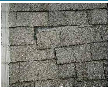
Problem: Slipping shingles. Shingles can slip when the manufacturer's fastening instructions are not followed. Improper practices include using too few fasteners, and overdriving and underdriving the fasteners. Solution: Follow the shingle manufacturer's fastening instructions as printed on the bundle wrappers.
