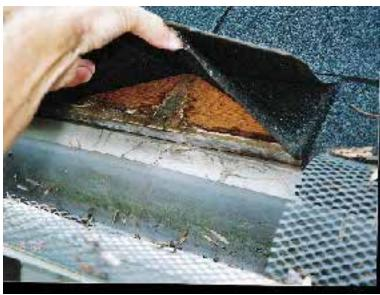
Problem: Felt underlayment incorrectly lapped under (instead of over) the metal drip edge. Any water that may get under the shingles — for instance, from wind-driven rain — should be carried by the felt underlayment over the top of the drip edge. Solution: Lap the felt underlayment over the drip edge.
