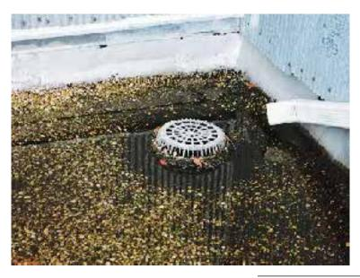
**Problem:** Clogged roof drain. Failure to clear away leaves from a drain strainer can cause ponding.
