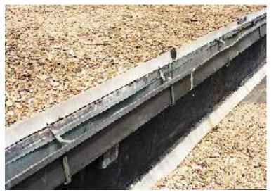
Problem: Edge flashing was not nailed. The installer forgot to attach the edge flashing to the roof before the built-up roofing was installed. When the roofing material later contracted, it pulled the entire flashing away from the edge of the roof.
