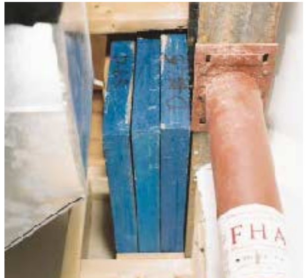
Figure 1. To make space for a downstairs family room, the author recently removed a column under a main steel girder and sistered a triple LVL to the girder to carry the span. An engineer provided the design.
