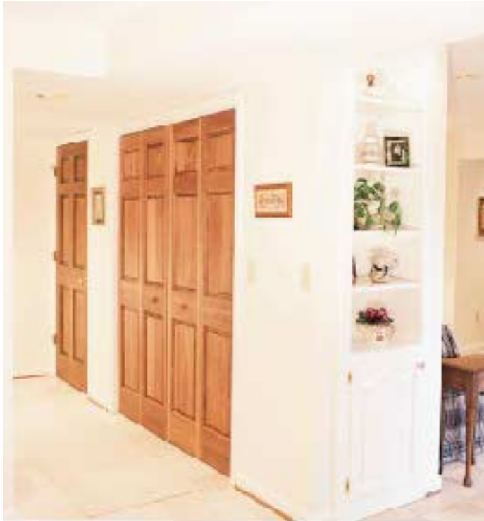
Figure 5. The angled table built into the corner disguises this home’s water supply shutoff valve. Access is through the top.
