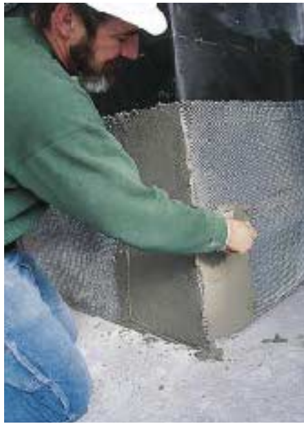
Figure 4. Like a stucco installation, manufactured stone is installed over a water-resistant paper and galvanized lath (left). A scratch coat (right) provides the flat surface for setting the stone.
