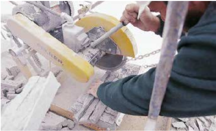
Figure 5. Manmade stone can be cut with the usual mason's tools, like diamond-blade saws (above) and grinders (right).
