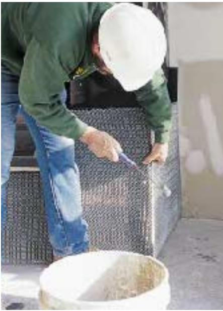
Figure 4. Like a stucco installation, manufactured stone is installed over a water-resistant paper and galvanized lath (left). A scratch coat (right) provides the flat surface for setting the stone.
