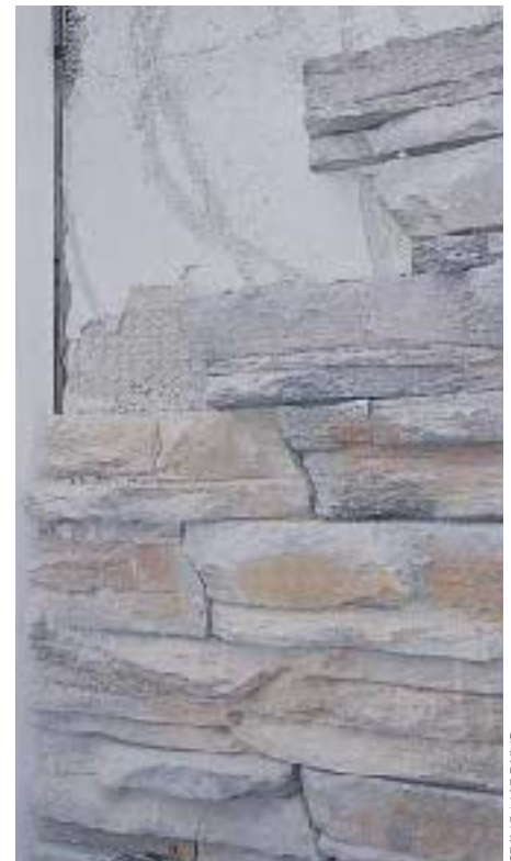
Figure 1. Installation details for manufactured stone resemble those of three-coat stucco. The photo shows stone mounted on a scratch coat in diamond lath. The product typically adds about 12 psf to the weight of the wall.
