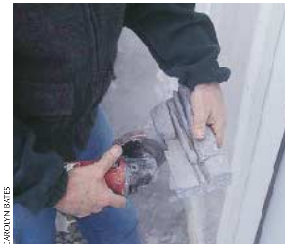
Figure 5. Manmade stone can be cut with the usual mason's tools, like diamond-blade saws (above) and grinders (right).
