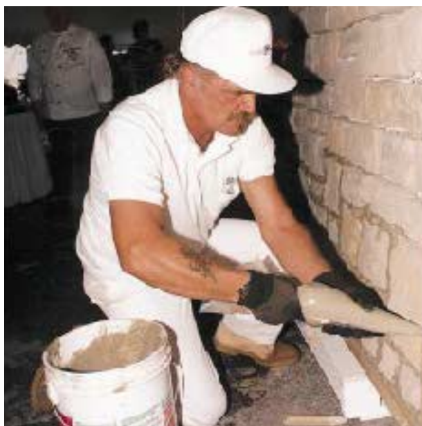
Figure 6. Grout is installed with a grout bag. Drystack stone styles require no grouting, except perhaps to fill small voids.
