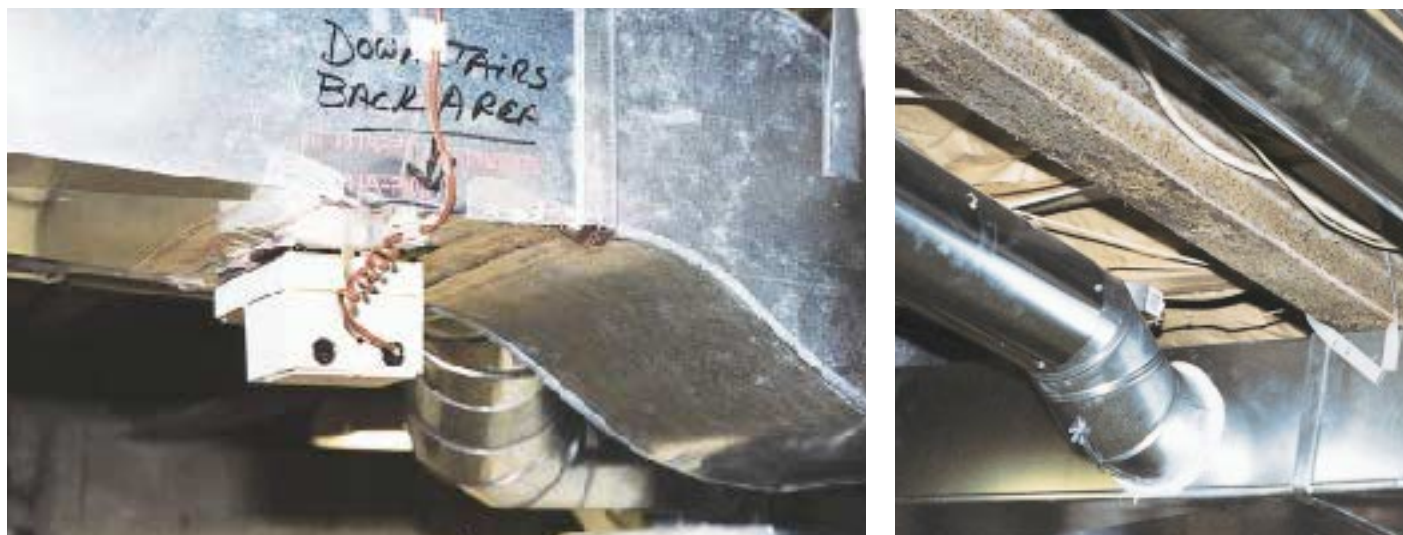
Figure 2. Rectangular motorized dampers are placed near the furnace (left); round dampers for branch ducts are located as close to the trunk lines as possible (right).
