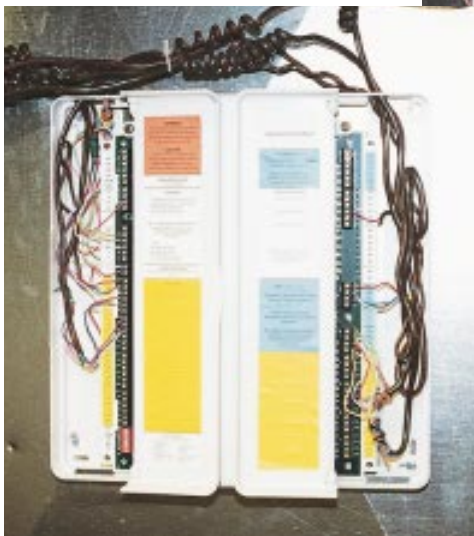
Figure 3. The author connects wiring from dampers and thermostats at the furnace-mounted control panel. Standardized electronic circuitry in the more sophisticated zone control panels makes even complicated zone designs easy to troubleshoot.
