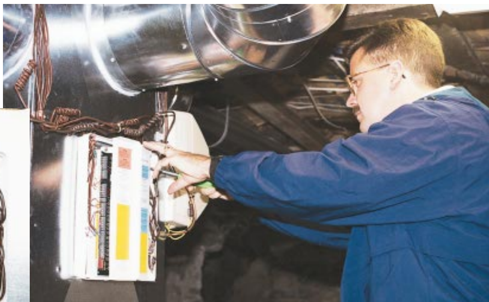
Figure 3. The author connects wiring from dampers and thermostats at the furnace-mounted control panel. Standardized electronic circuitry in the more sophisticated zone control panels makes even complicated zone designs easy to troubleshoot.
