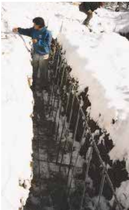
Figure 5. A sudden snow storm the day after the pour delayed foundation work, but workers were back in the trench 24 hours later. The lean fill kept melting snow from turning the trench into a mud hole.
