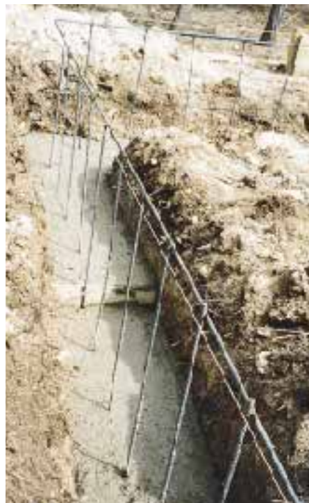
Figure 6. Structural footing concrete was placed on top of the lean fill within a week. For heavy structural loads, check with an engineer to see if the lean fill will have to cure longer than seven days.
