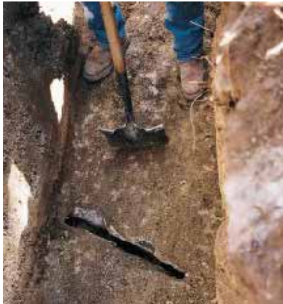
Figure 1. Lean fill was a simple way to consolidate the loose rock and span or fill the numerous fissures — some as wide as 2 inches — that crisscrossed the irregular bedrock.
