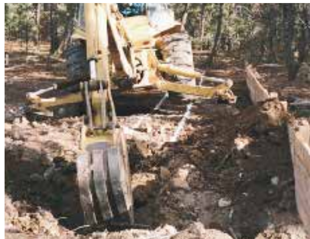
Figure 4. Trenches for the footings were dug with a backhoe, following lines marked on the ground. To avoid loosening the fractured bedrock, the operator was careful to keep the bucket teeth from snagging.
