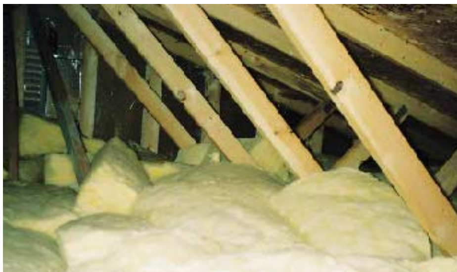
Figure 8. Sloppy batt installation, and a thermal canyon excavated by the electrician. You get what you inspect , not what you expect .
