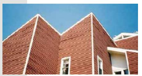
The clapboard siding on this building has no roof protection. It is curling and splitting, and requires repainting every three years.
