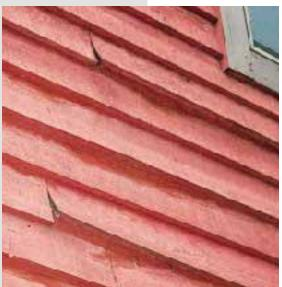
Locate clapboard siding joints over studs so that the nails penetrate the framing.
