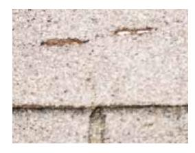
Protruding fasteners can cause breaks in asphalt shingles.
