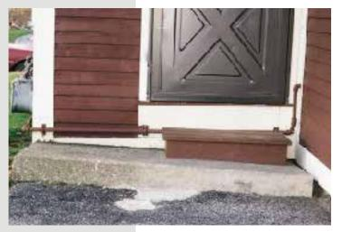
This wooden step (above) was built to compensate for a concrete stoop that settled. The photo at right shows how a settling patio slab directs rainwater toward the house.
