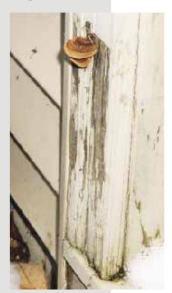
When an exterior door has no roof protection, the lower sections of the jambs and door are vulnerable to rot or rust.
