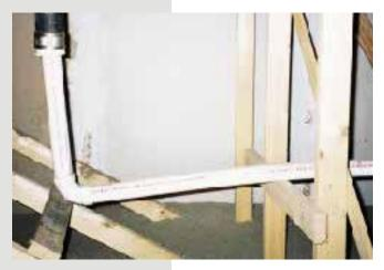
Most plumbing codes require horizontal lengths of plastic pipe, including vent pipe, to be supported every 4 feet. It is especially important to install a pipe hanger near the point where the vent turns to penetrate the roof.
