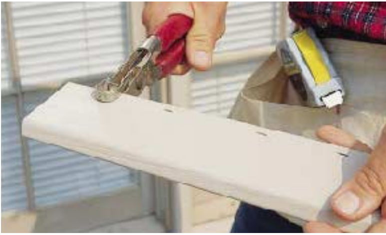
Figure 9. A snap-lock punch creates small lugs in the edge of the siding. These lugs keep the siding in place when it is slid into undersill finish trim.
