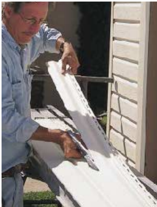
Figure 10. Vinyl siding can be cut with shears (right) or a circular saw (below). When using a circular saw, a fine-toothed plywood blade is used, inserted backwards.
