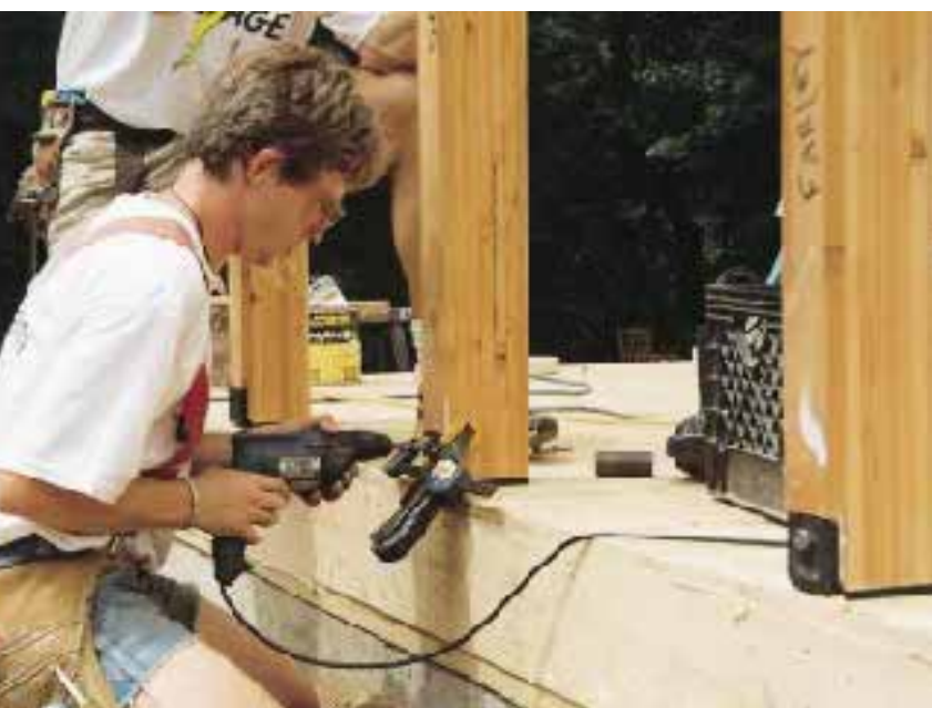
Figure 1. Steel beam shoes bolted to solid blocking and to the notched faces of the columns fix the sunroom frame to the deck.
