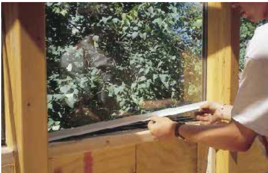
Figure 13. Lengths of aluminum angle, caulked to the kneewall sill, provide weep gutters that prevent condensation from pooling on the finished sill.
