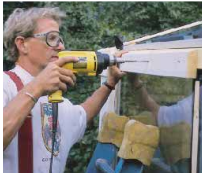
Figure 9. Angled blocking screwed to the eaves purlin secures the glass and directs condensation away from the vertical glass.
