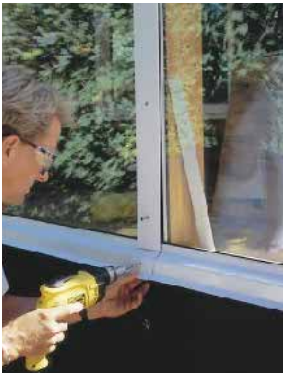
Figure 10. Stainless steel screws secure seam cover pieces that overlap adjoining sections of kickout flashing. Aluminum battens backed with glazing tape seal IGUs solidly to the glulam frame.
