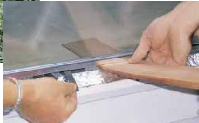
Figure 8. Rubber glazing-blocks support vertical IGUs where they rest on the kneewall top plate. Wooden shims are useful for aligning blocks.
