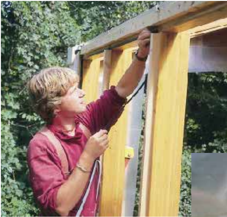
Figure 7. Pine spacers nailed to beams define “pockets” sized for insulated glass units. Vinyl foam glazing-tape is applied to the glulam frame to act as a seal between the frame and IGUs.
