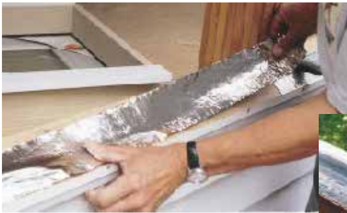
Figure 5. Foil-faced butyl tape is applied to the kneewall top plate (above) and the eaves purlin (right) to shed condensation. Aluminum angle-glazing supports and vinyl weep gutters are also mounted on the eaves purlin.
