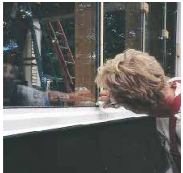
Figure 12. Silicone caulk provides a final seal against rain and meltwater. The author applies a liberal bead of caulk (top), before using an empty caulk tube to scoop up the excess and leave a uniform profile (above).
