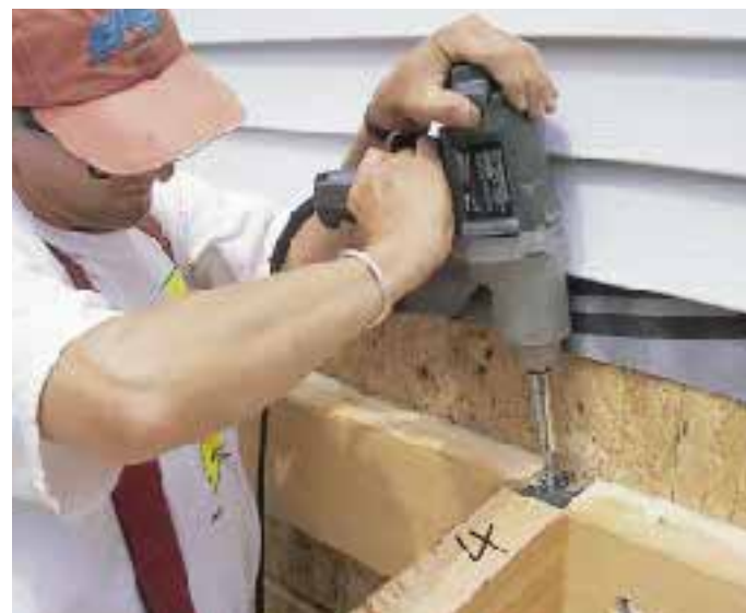
Figure 2. After bolting the prefabricated ledger board to the house wall (top left), the crew erects glulam column and rafter units (top right). Custom beam hangers, attached to the rafter ends, drop into slots routed into the ledger (above), providing a strong, totally concealed connection.
