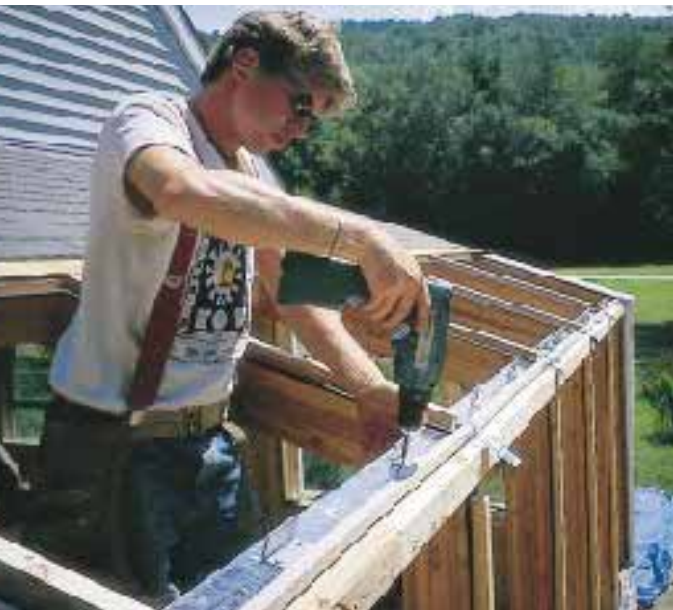
Figure 6. A slight crown in the centers of the weep gutters on the eaves purlin prevents condensation from pooling within. The foil overlaps the lower lip of the weep gutter, acting as flashing to direct condensed moisture into gutters.
