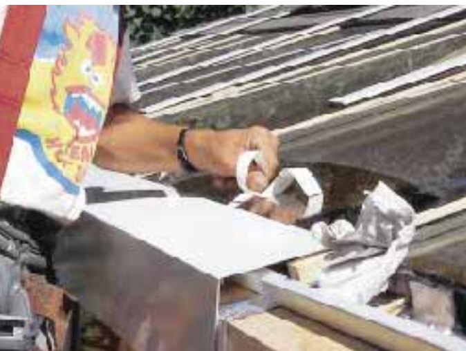
Figure 11. Two-sided sticky tape secures transition flashing to glass units at the eaves. Pressure from aluminum battens applied later will lock them solidly in place.
