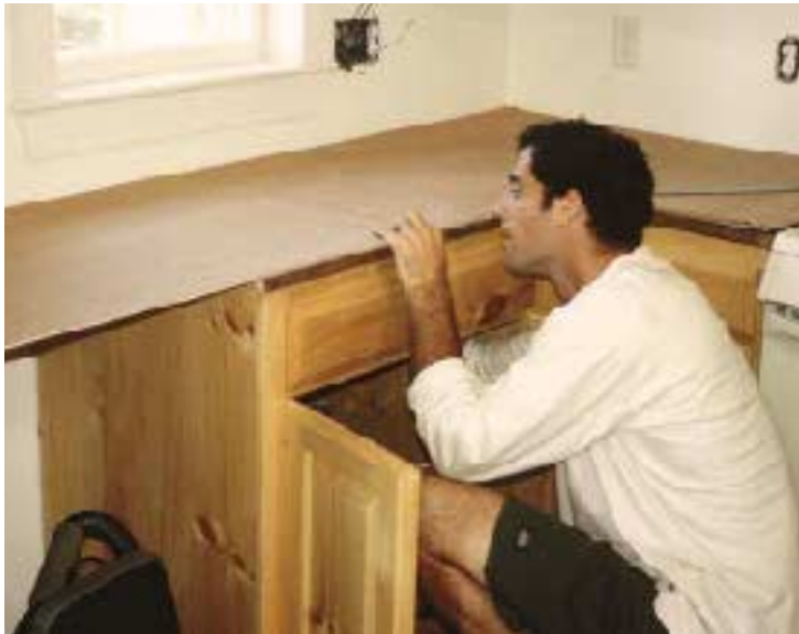
Figure 2. Lauan plywood templates, cut to the final outline of the countertops, precisely copy the site conditions and direct the shaping of the casting forms. The author traces a spacer block to establish the cut line of an edge overhang.
