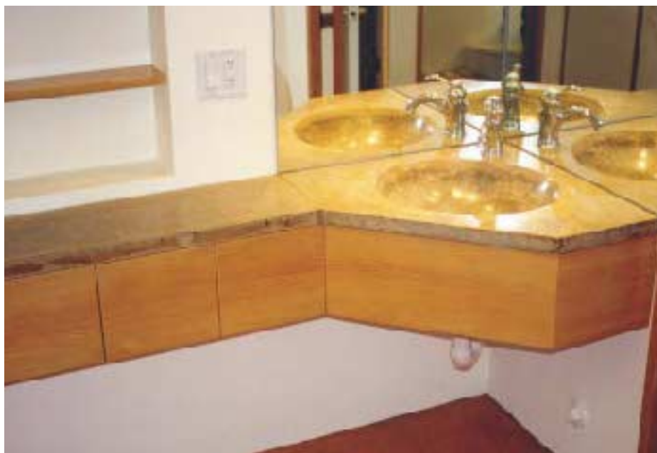
Figure 1. Prefabricating cast concrete makes it possible to create compound shapes and incorporate something as complex as a custom integral sink basin into a countertop.
