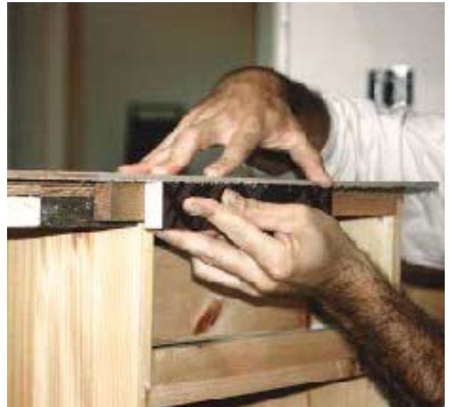
Figure 2. Lauan plywood templates, cut to the final outline of the countertops, precisely copy the site conditions and direct the shaping of the casting forms. The author traces a spacer block to establish the cut line of an edge overhang.
