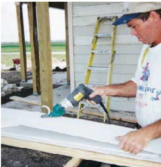
Figure 1. The SS304 Snapper Shear will cruise through miles of siding between blade changes, and it's dust free (left). The new Model 6604 shears from Porter-Cable are especially easy to handle, and the belt clip is handy (right).
