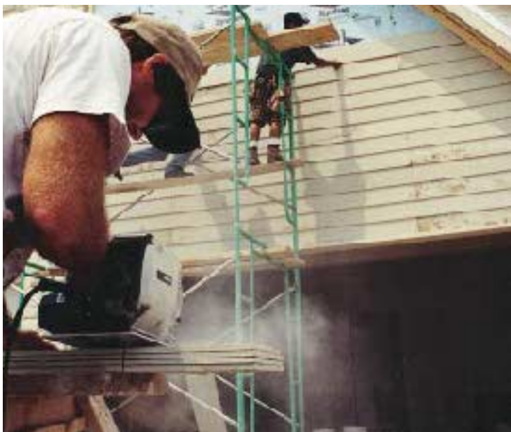
Figure 5. By themselves, the dust collectors on these saws don't completely eliminate the dust, but they do cut it down. If you hook up a vacuum, however, they are just about dust-free.
