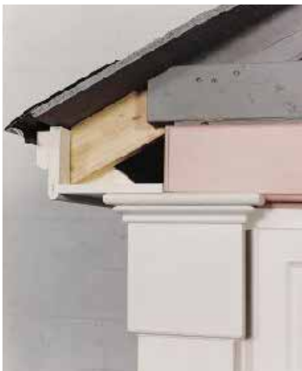
Figure 5. Cellular PVC is a type of vinyl that has been foamed and extruded. It is weather-resistant, even if left unpainted.
