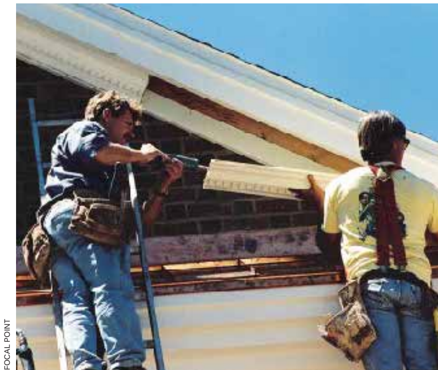
Figure 4. Because polyurethane trim, also called polymer trim, is molded, not extruded, complicated profiles like dentils are possible. It can be cut and machined like wood (left), and is installed with adhesive (above).
