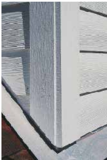
Figure 3. This Harditrim HLD, like Cemtrim, is a low-density fiber-cement product. Low-density fiber-cement trims can be installed proud of the siding without the shimming required for thinner fiber-cement trim boards.
