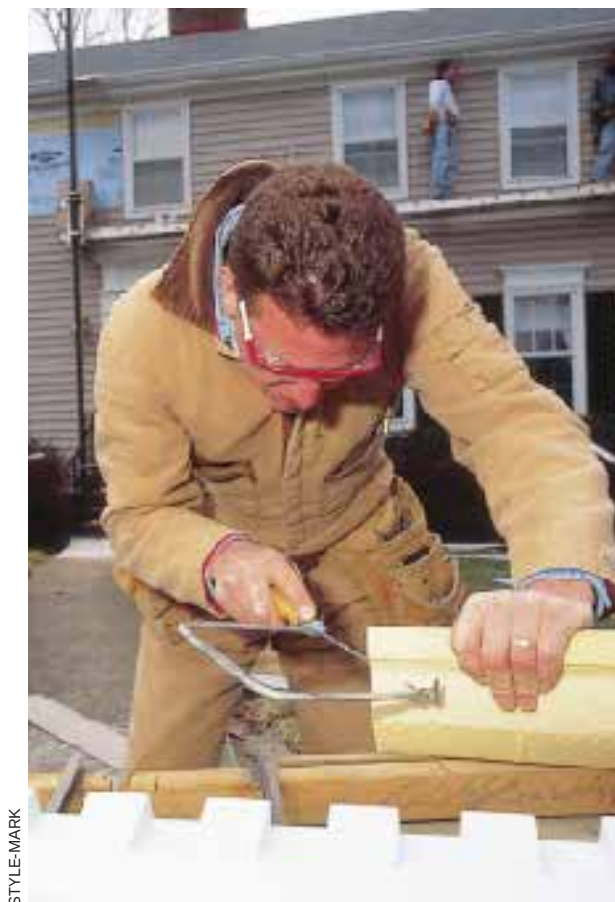
Figure 4. Because polyurethane trim, also called polymer trim, is molded, not extruded, complicated profiles like dentils are possible. It can be cut and machined like wood (left), and is installed with adhesive (above).
