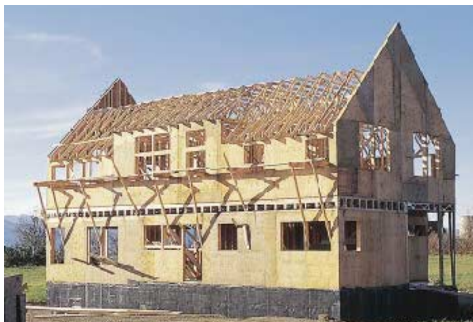
Figure 5. The top half of the piggyback trusses went up next (above). The shed dormer houses the master and guest bathrooms. At left, the nearly finished house.
