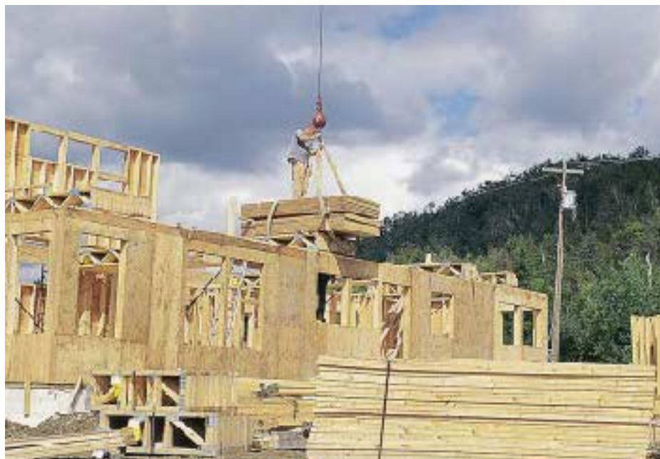
Figure 2. Bundled second-floor trusses are set atop the first-floor walls. The lumberyard strapped together several sheets of plywood subfloor before delivering it to the job site. The 20-foot-high stairwell panels are visible in the background.
