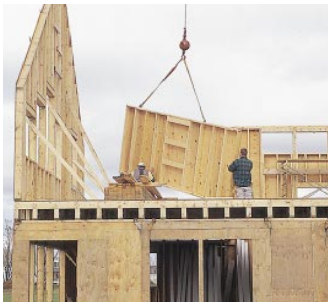
Figure 4. Second-floor exterior wall panels were lifted individually into place from the ground. The gable wall panels were framed floor to roof as single units to avoid a potential hinge effect that might arise with separate wall and gable panels.
