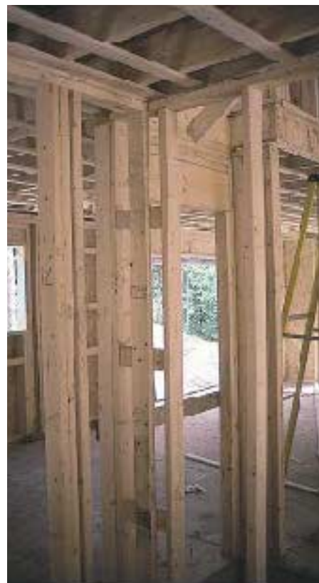
Figure 3. Partition-wall intersections are simplified by the presence of framing “ladders.” The end stud of the adjoining wall is nailed to the ladder, as shown here, making it easy to adjust the final position of non-bearing partitions as needed.
