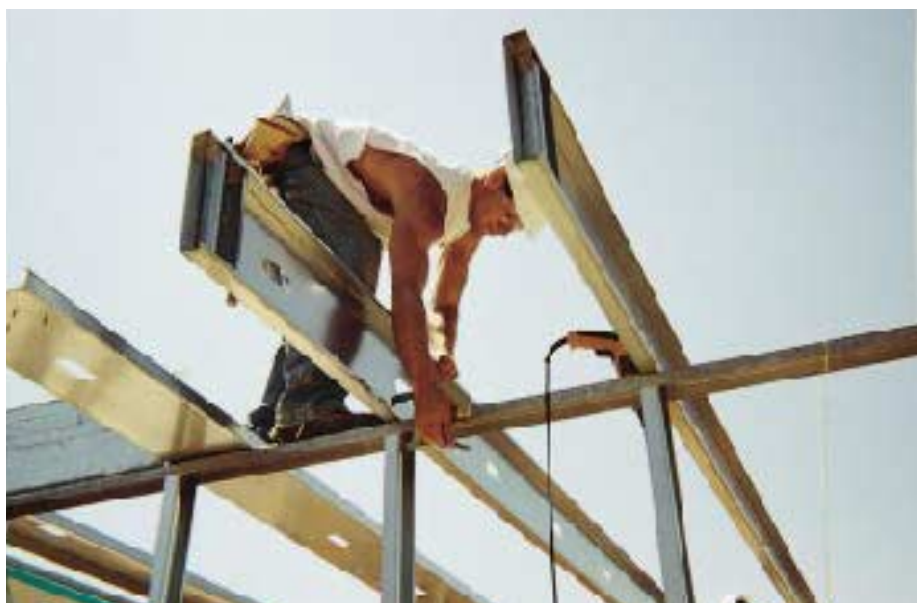
Figure 8. A framer clamps the cantilevered floor joist to the top track before screwing it in place. Additional web stiffeners will be added where the joists bear on the plate. Floor cantilevers of up to 2 feet are permitted by the prescriptive method.
