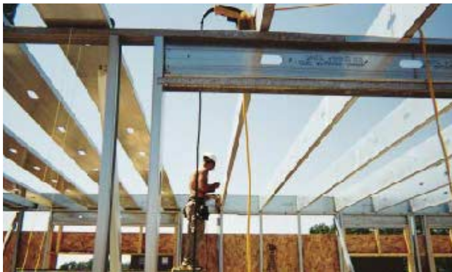
Figure 7. Second-floor joists are fastened to the top track of a steel-framed wall with screws driven through the joist flanges. OSB sheathing will be screwed to both studs and rim track for a secure connection between floor and wall framing.
