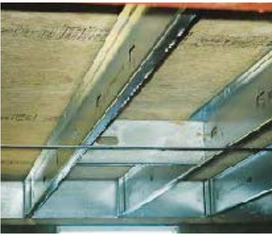
Figure 10. Joists are braced with 1 1/2 inch steel strapping at mid span, and spaced blocking fastened to the joists with clip angles.
