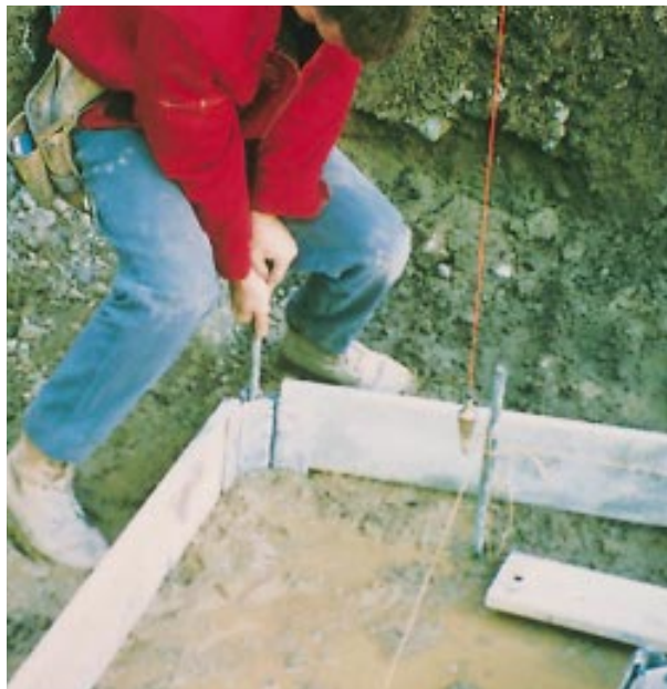
Figure 5. If a form stake sinks in too easily, the soil may be too soft. For localized soft spots, the author recommends widening the footing. In wet, mucky areas, he recommends compacting large cobbles into the mud to provide bearing.
