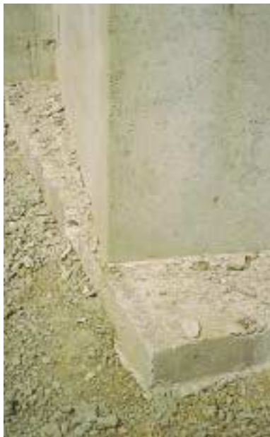
Figure 3. This incorrectly placed footing caused the foundation wall to be off-center. If the soil is very strong, this may not lead to problems. If the footing is on a weaker soil however, the author will recommend that it be fixed.
