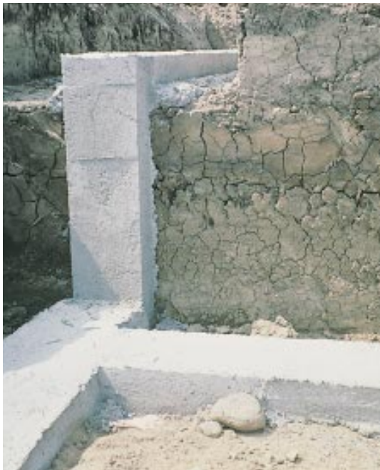
Figure 9. Stepped footings are used at changes in elevation in masonry foundations, but may not be necessary for poured concrete foundations.
