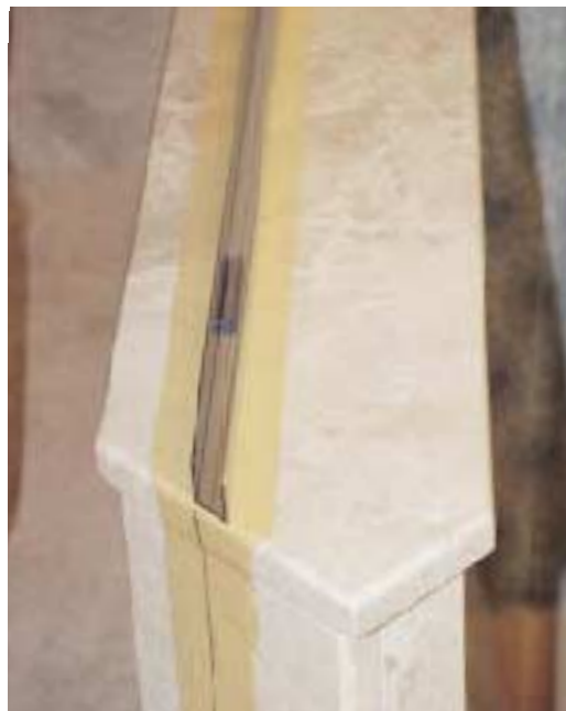
Figure 4. Masking tape provides a legible base for marking the layout line, locating transitions, hardware, and termination points, as well as quick line removal. Clear plastic setting blocks are positioned over the countersunk screw heads in the U-channel to protect the vulnerable edge of the tempered glass panel from contact with the metal and tiles.
