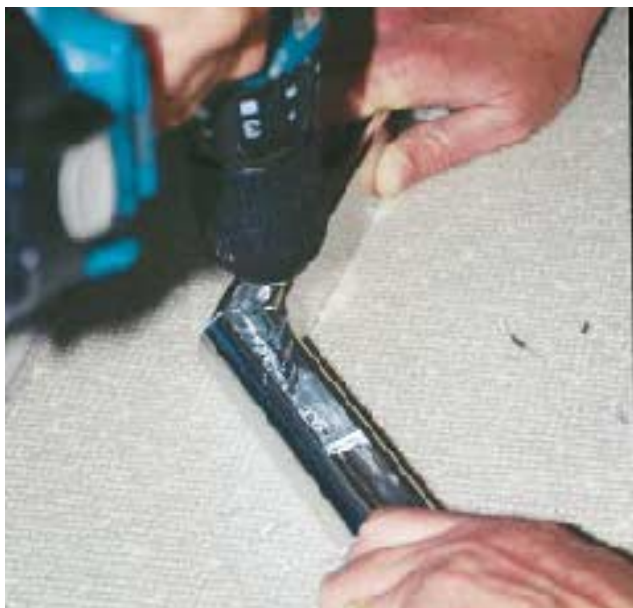
Figure 1. Head channel joining plates for frameless enclosures come in fixed corners of 90- and 135-degrees (left). Off-angles, which drive the cost of an enclosure up, are handled with an adjustable corner (above). The authors measure, cut, and join the extruded header sections on site.
