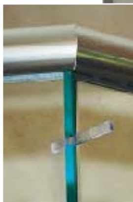
Figure 5. Trial assembly ensures that all of the components are positioned correctly, and that the door will operate freely, with the minimum necessary clearance to reduce water escape (above). With the header secured, the authors adjust and shim the door (right), using 1/8-inch-thick setting blocks to temporarily set the clearance gap (right, inset).
