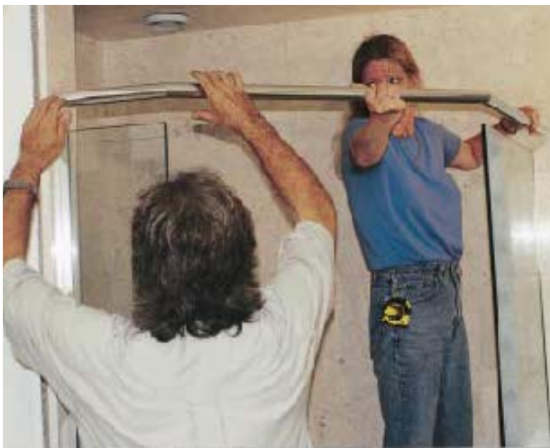
Figure 5. Trial assembly ensures that all of the components are positioned correctly, and that the door will operate freely, with the minimum necessary clearance to reduce water escape (above). With the header secured, the authors adjust and shim the door (right), using 1/8-inch-thick setting blocks to temporarily set the clearance gap (right, inset).
