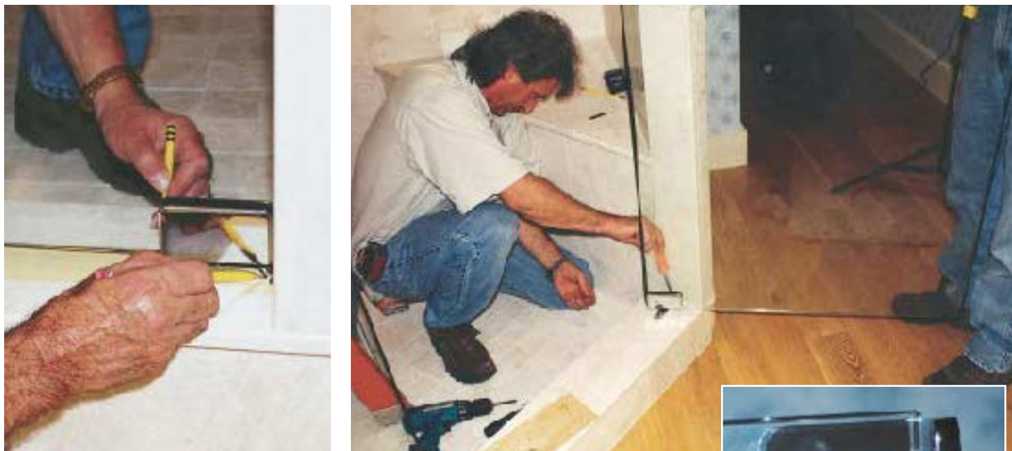
Figure 6. With the door gapped and shimmed, the authors trace the hinge location onto the threshold (above, left). It's difficult to completely seal a frameless enclosure, especially if the client doesn't like the look of the polycarbonate seals and edge wipes. The authors emphasize that wood floors and frameless enclosures make poor bathmates. Delicately handling heavy glass panels is always a two-person job (above, right). With the side panels permanently set and caulked, the pivot hinges can be secured and final-adjusted. Clearance around the hinge body allows minor adjustments to be made in the door's position (right).
