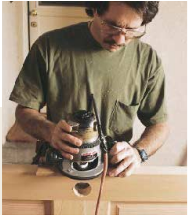
Figure 2. A shop-made template (above, left) and a router (above, right) are the tools of choice for mortising the latch. The author finishes the job with a corner chisel (left).
