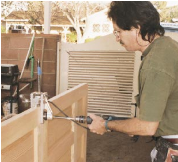
Figure 1. A lock boring jig ensures accurate hole placement. The author always drills the face bore first (above), then the edge bore (right).
