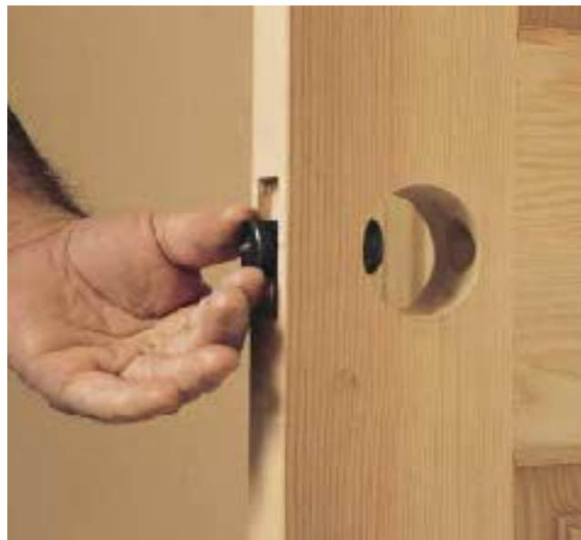
Figure 3. A center marker works well for quickly locating the lock strike, but is not entirely accurate.
