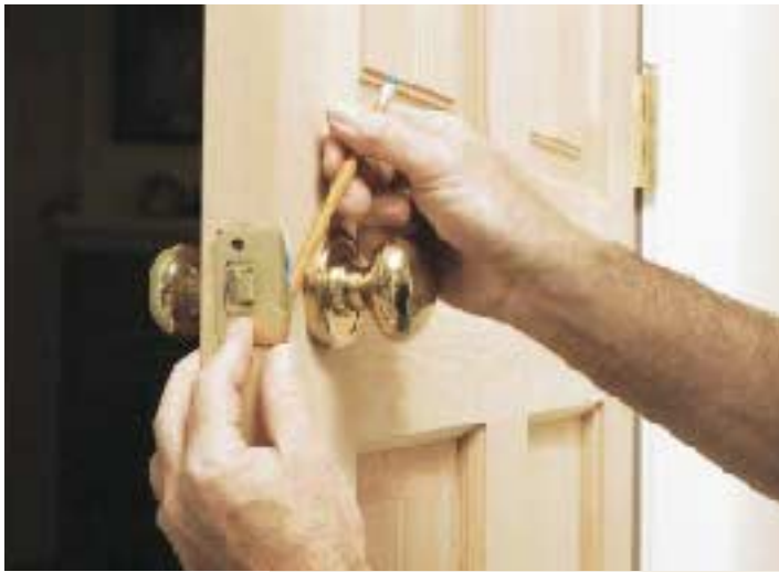
Figure 4. Holding the strike plate over the latch (above, left), the author marks the edge of the door onto a piece of masking tape placed on the back of the strike plate. He then closes the door and marks the centerline of the strike by eye (above, right), extending this line horizontally across the jamb. The author then lines up the vertical line on the tape with the edge of the door, centering the strike hole over the horizontal line (right) to lay out the strike plate mortise.
