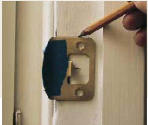
Figure 4. Holding the strike plate over the latch (above, left), the author marks the edge of the door onto a piece of masking tape placed on the back of the strike plate. He then closes the door and marks the centerline of the strike by eye (above, right), extending this line horizontally across the jamb. The author then lines up the vertical line on the tape with the edge of the door, centering the strike hole over the horizontal line (right) to lay out the strike plate mortise.
