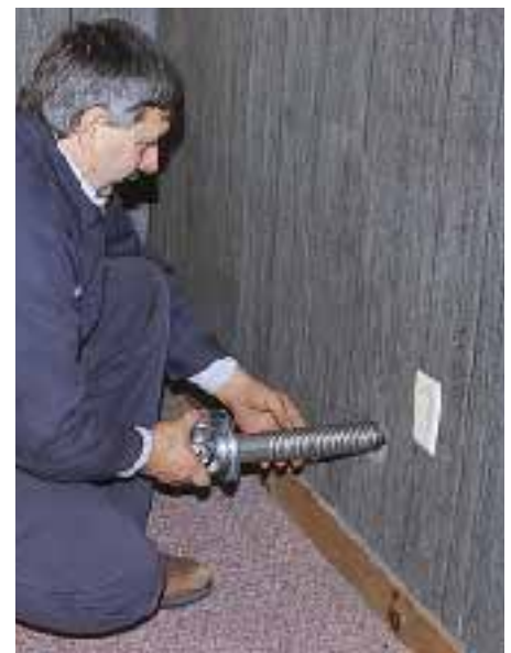
Figure 4. A cardboard installation template locates the vent pipe and fuel line holes. Before drilling the 2½-inch hole for the vent pipe, check for wiring, plumbing, and other obstructions by first drilling a small hole. The vent pipe assembly consists of two concentric pipes — a smaller vent pipe inside the larger air intake pipe.
