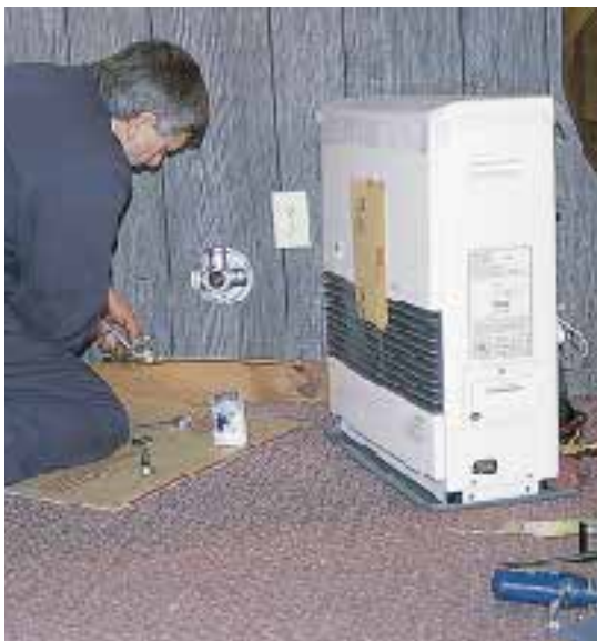
Figure 6. A Firomatic safety valve, which shuts down the flow of fuel in the event of a fire, is installed in the ¾-inch copper fuel line behind the heater. The flexible air intake pipe (foreground, right-hand photo) is installed between the heater and the stainless steel vent pipe assembly.
