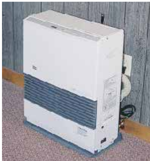
Figure 1. Direct-vent heaters are very compact, making them good choices for small houses without basements or utility rooms.
