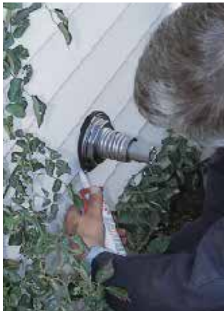
Figure 5. The sidewall vent terminations for the Rinnai and Monitor heaters are made of stainless steel. These fittings are equipped with a rubber boot that can conform to the irregular profiles of a wide variety of siding types, including clapboard. Some installers caulk the joint between the siding and the vent termination boot.
