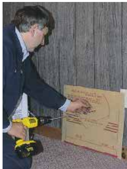
Figure 4. A cardboard installation template locates the vent pipe and fuel line holes. Before drilling the 2½-inch hole for the vent pipe, check for wiring, plumbing, and other obstructions by first drilling a small hole. The vent pipe assembly consists of two concentric pipes — a smaller vent pipe inside the larger air intake pipe.
