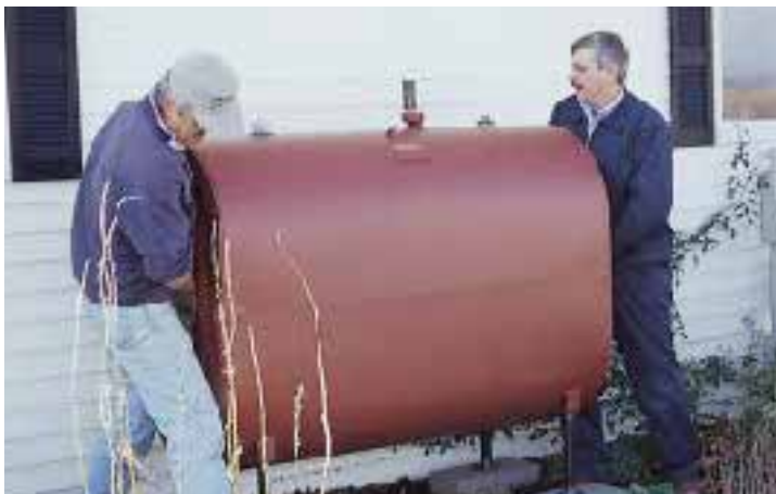
Figure 2. The kerosene tank is best located on the north side of a house, where it is shaded from high temperatures. The tank must be installed on either concrete blocks or a slab, depending on local codes. In any case, it must be level (right).
