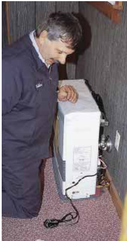
Figure 6. A Firomatic safety valve, which shuts down the flow of fuel in the event of a fire, is installed in the ¾-inch copper fuel line behind the heater. The flexible air intake pipe (foreground, right-hand photo) is installed between the heater and the stainless steel vent pipe assembly.
