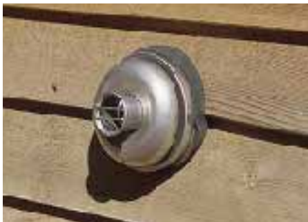
Figure 5. The sidewall vent terminations for the Rinnai and Monitor heaters are made of stainless steel. These fittings are equipped with a rubber boot that can conform to the irregular profiles of a wide variety of siding types, including clapboard. Some installers caulk the joint between the siding and the vent termination boot.
