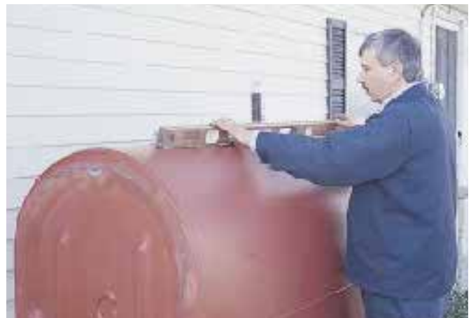
Figure 2. The kerosene tank is best located on the north side of a house, where it is shaded from high temperatures. The tank must be installed on either concrete blocks or a slab, depending on local codes. In any case, it must be level (right).
