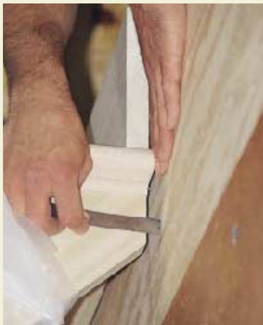
Figure 11. A \frac{5}{8} -inch gap is left for installing drywall around the stairs (right). Precut shims (far right) speed this process.
