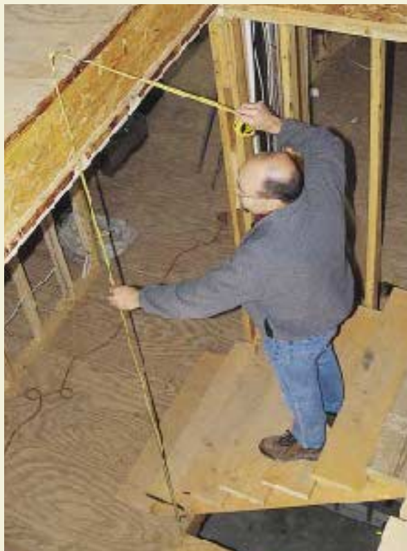
Figure 2. Stairbuilders will quote jobs from plans, but they generally send a field rep to the site to verify measurements before starting work.
