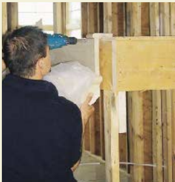
Figure 7. Two men can easily carry and place a typical straight staircase (left). For large or complicated staircases, you may need more manpower. The installer pins the lower staircase section in place, using a scrap of landing tread to determine the correct height for the top edge of the riser (right). He places the first screw where cove molding will cover it later.
