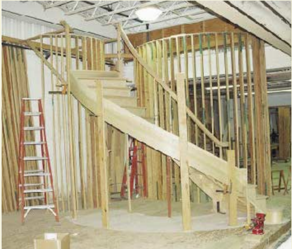
Figure 1. Curved stairs are built on a wall mockup that is framed using plates cut from a full-scale CAD pattern. Identical plates are sent to the site so the actual wall will match the shop jig. Railings are test-fitted in the shop before the stair is shipped.
