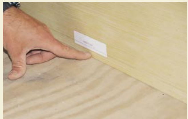
Figure 9. The installer uses a piece of landing tread, supplied with the stairs, to check the fit at the top (left). A label on the lowest riser (above) shows the finish floor height and indicates the centerline of the stairs.
