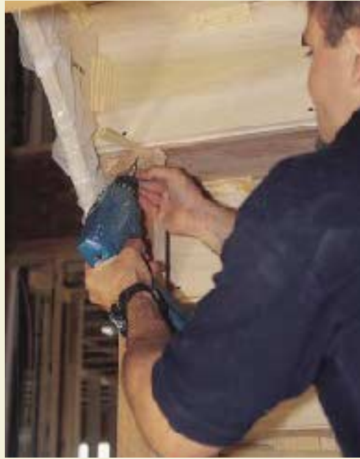
Figure 12. Before leaving, the stair installer places temporary braces at mid-span in each run of stairs. It's best to build in a crown of perhaps \frac{1}{4} inch to allow for slight settling and framing lumber shrinkage over time.
