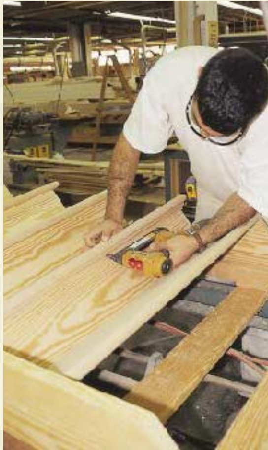
Figure 5. Glue blocks are stapled and glued to every joint from the underside (far left) to add solidity and prevent squeaks. Next, cove molding is finish nailed beneath each tread nosing (left).
