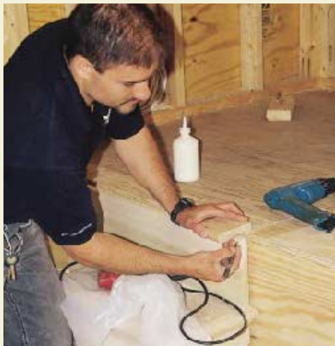
Figure 9. The installer uses a piece of landing tread, supplied with the stairs, to check the fit at the top (left). A label on the lowest riser (above) shows the finish floor height and indicates the centerline of the stairs.
