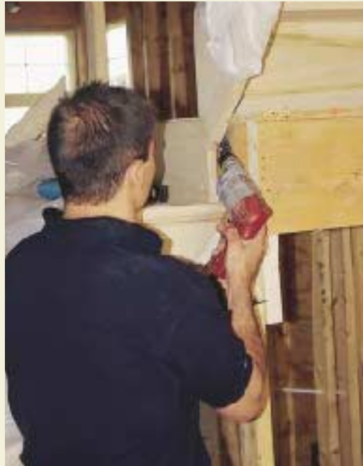
Figure 8. The joint at the landing newel (far left) serves as a focal point for aligning the entire stair assembly. The installer shims and plumbs this location carefully, then screws through the upper stair stringer into the lower stair riser to firmly lock the joint (left). Fasteners at this point will be covered later by the newel-post.
