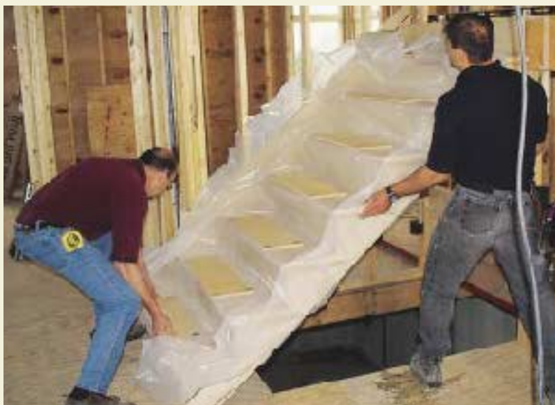
Figure 7. Two men can easily carry and place a typical straight staircase (left). For large or complicated staircases, you may need more manpower. The installer pins the lower staircase section in place, using a scrap of landing tread to determine the correct height for the top edge of the riser (right). He places the first screw where cove molding will cover it later.
