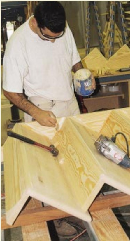
Figure 4. Stringers are precision-routed on a computer-controlled machine. The treads are securely wedged (left), glued (center), and screwed (right) in place.
