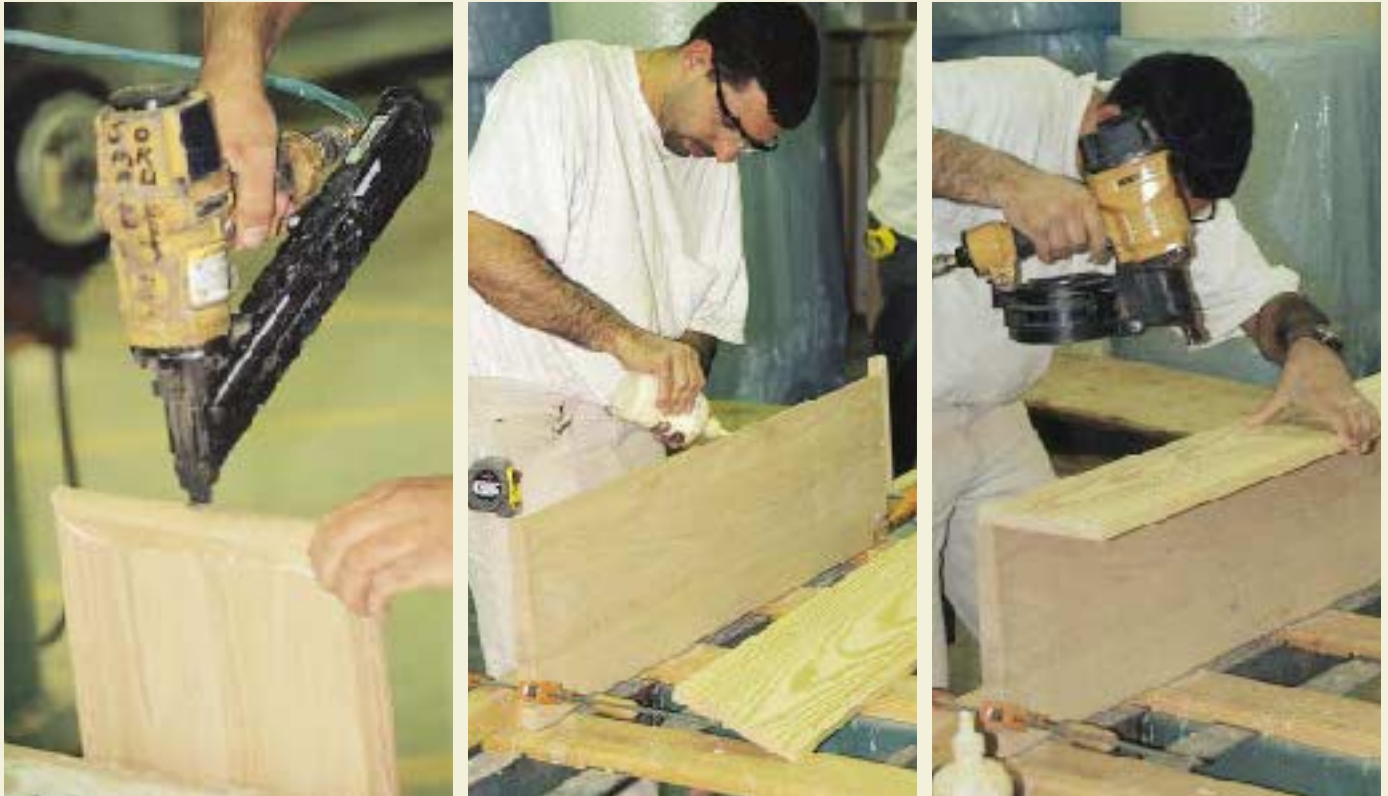
Figure 3. Perfect-fitting tread returns are glued and air-nailed to the treads (left). A tongue on the back of each tread (center) matches a groove routed into the face of each riser. Gluing and nailing these joints, the stair builder makes up a complete set of tread-riser pairs in about 20 minutes (right).
