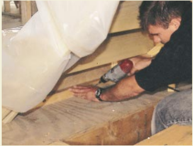
Figure 10. A cleat glued and screwed to the deck serves to hold the bottom stringer tight to the floor (right). Screws into the cleat through the face of the stringer will be buried behind flooring and molding. Screws into the studs from underneath are also invisible (below, left). Visible fasteners (below, right) are counter sunk and plugged.
