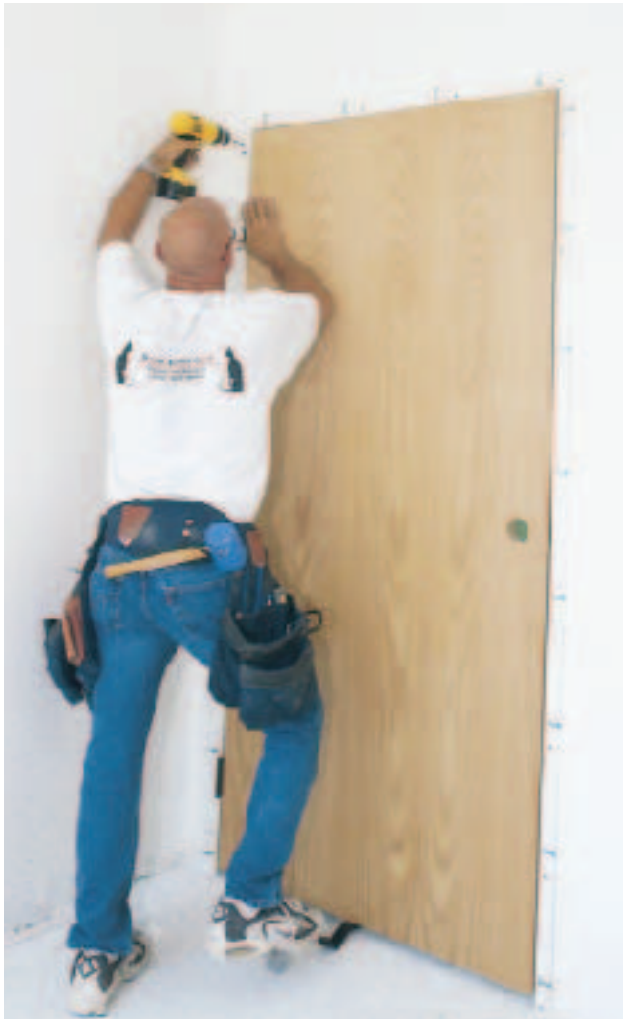
Figure 5. Control the head gap by stepping on a pry bar slipped under the door, then drive a screw into the top hole in the hinge jamb (left). Drive another screw through one of the holes beneath the bottom hinge (above), then check the jamb for plumb. Finally, correct the gap at the strike jamb by pressing harder on the bar while driving an additional screw behind the top hinge (below).
