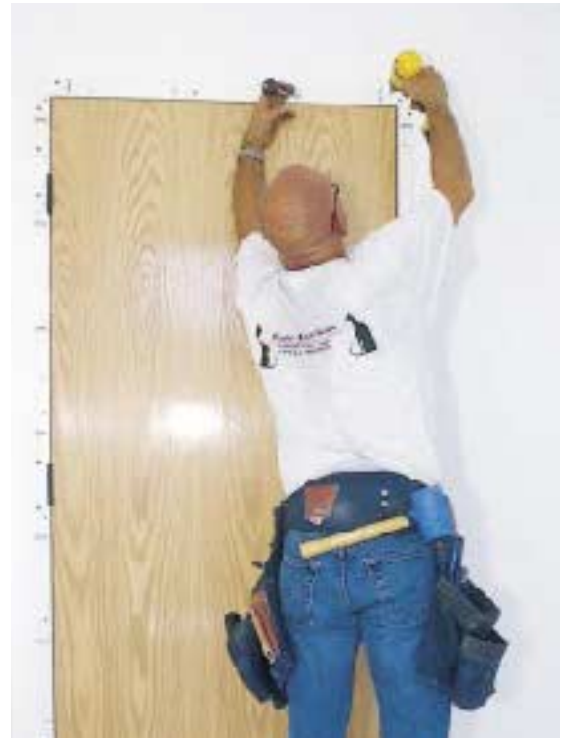
Figure 6. If necessary, correct the head gap by giving the strike jamb an upward shove with the pry bar before driving a screw through its top (left). To ensure a tight corner joint, use an awl to pull the head jamb downward before screwing the end into place (above). Starting at the top of the strike jamb, drive a screw every 12 inches or so, adjusting the strike gap with the awl as needed (below).
