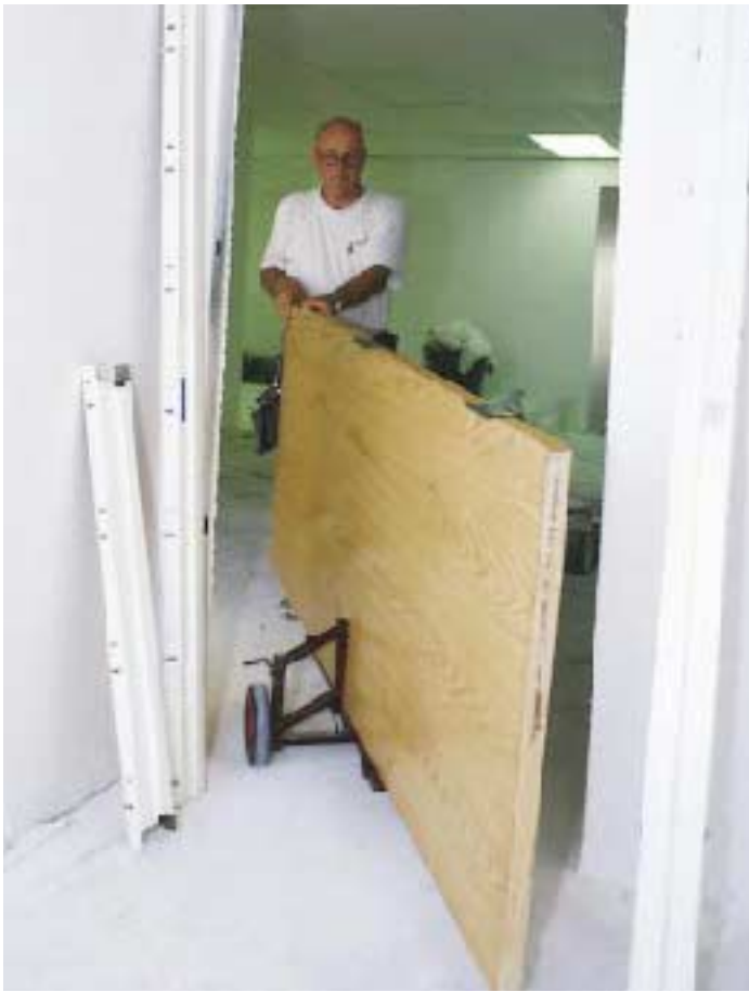
Figure 1. A dolly makes it easy to move doors on site (left), and also supports them while hinges are installed (right). It's convenient to use two cordless drills for this task — one with a Vix bit and the other with a Phillips bit.
