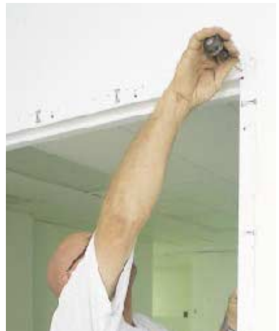
Figure 3. Use an awl to pry the head jamb downward, eliminating any gaps between the head and side jambs.
