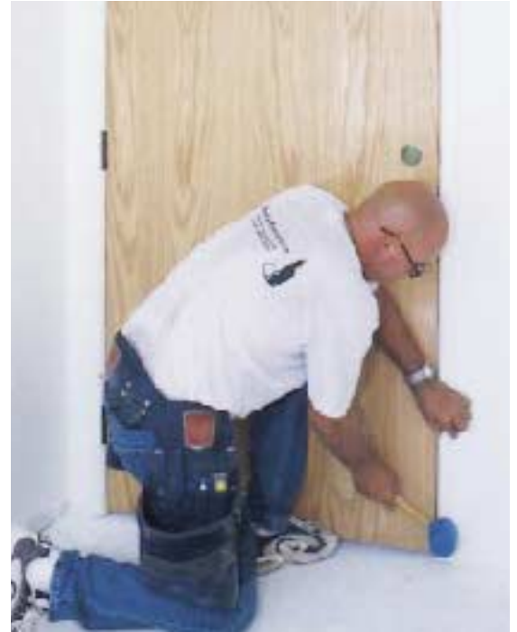
Figure 7. Center the head casing, press it against the spring clips, and gently tap with a mallet to snap it home. Repeat for the legs, starting at the top miter joint and working downward.
