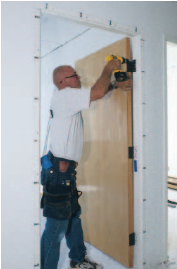
Figure 4. With the door turned 90 degrees to the opening, rock it forward onto the corner of the strike stile to align the top hinge leaf with the mortise, and secure it with a single screw (left). Bring the middle hinge into alignment by pushing the hinge stile with your foot, then secure the middle hinge with a second screw (below).
