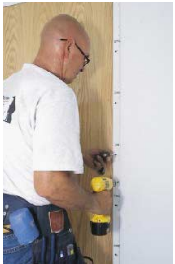
Figure 6. If necessary, correct the head gap by giving the strike jamb an upward shove with the pry bar before driving a screw through its top (left). To ensure a tight corner joint, use an awl to pull the head jamb downward before screwing the end into place (above). Starting at the top of the strike jamb, drive a screw every 12 inches or so, adjusting the strike gap with the awl as needed (below).
