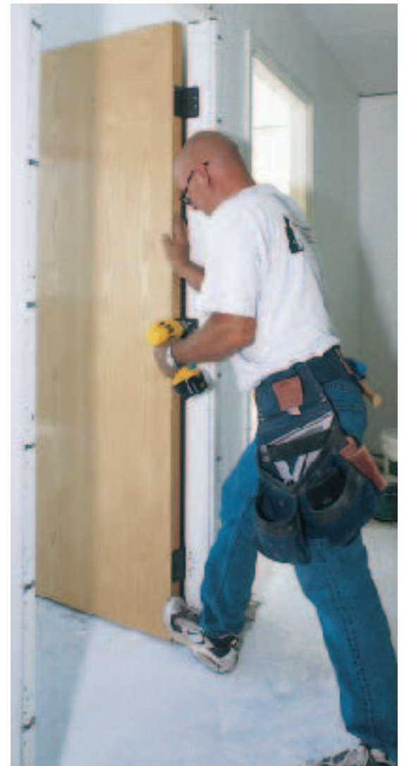
Figure 4. With the door turned 90 degrees to the opening, rock it forward onto the corner of the strike stile to align the top hinge leaf with the mortise, and secure it with a single screw (left). Bring the middle hinge into alignment by pushing the hinge stile with your foot, then secure the middle hinge with a second screw (below).
