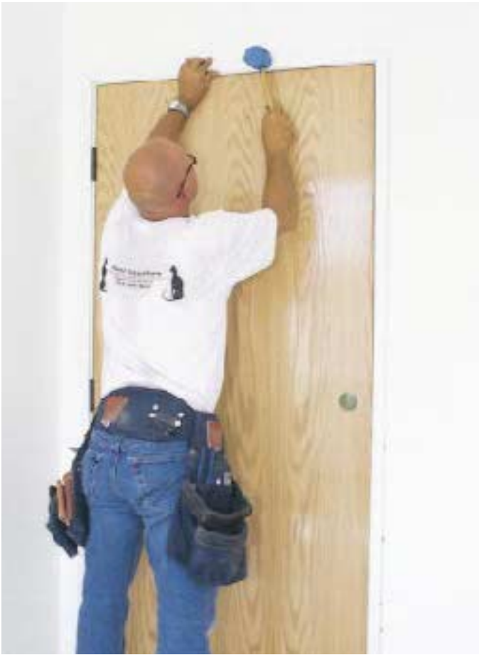
Figure 7. Center the head casing, press it against the spring clips, and gently tap with a mallet to snap it home. Repeat for the legs, starting at the top miter joint and working downward.
