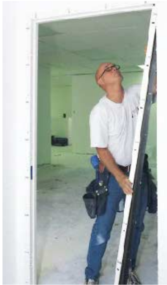
Figure 2. Installing a metal door jamb starts at the top: Slip the head jamb over the header (left), then angle the legs into the corners and push them into place (right).
