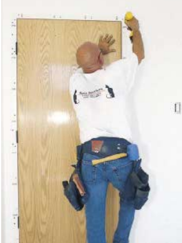
Figure 6. If necessary, correct the head gap by giving the strike jamb an upward shove with the pry bar before driving a screw through its top (left). To ensure a tight corner joint, use an awl to pull the head jamb downward before screwing the end into place (above). Starting at the top of the strike jamb, drive a screw every 12 inches or so, adjusting the strike gap with the awl as needed (below).
