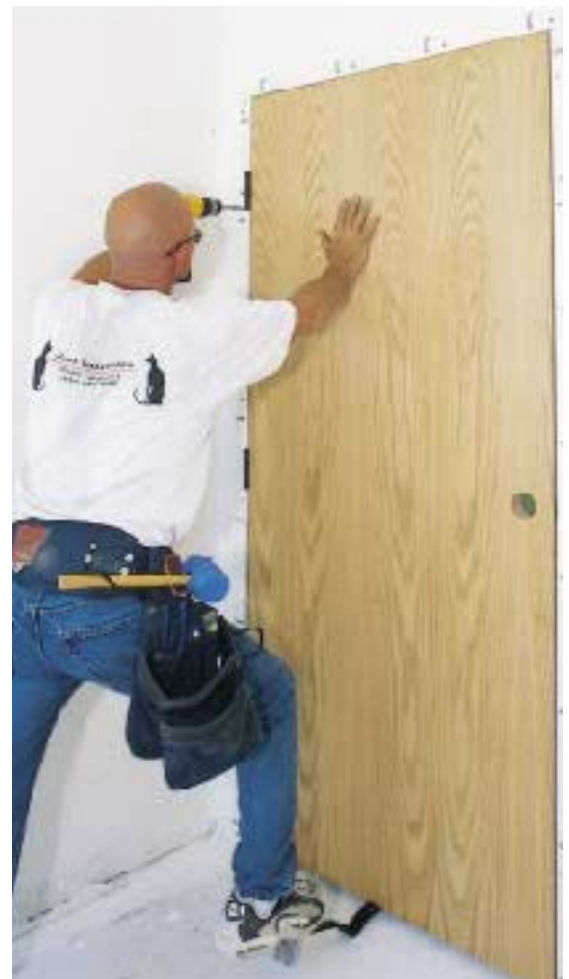
Figure 5. Control the head gap by stepping on a pry bar slipped under the door, then drive a screw into the top hole in the hinge jamb (left). Drive another screw through one of the holes beneath the bottom hinge (above), then check the jamb for plumb. Finally, correct the gap at the strike jamb by pressing harder on the bar while driving an additional screw behind the top hinge (below).
