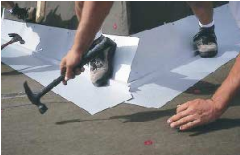
Figure 4. Where the tops of two valleys intersect a dormer ridge, one of the valleys is run past the intersection (left). Then the valley is carefully trimmed and folded to create a tight flashing (right). Use caulk at vulnerable corners.
