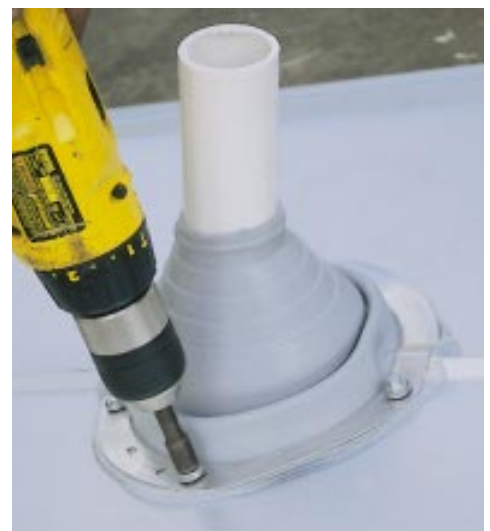
Figure 9. The best flashing for a plumbing vent is the Dektite boot. The boot is slipped over the pipe after the panel is installed. After installing a circle of caulk (left), the aluminum ring on the flashing is pressed down to conform to the ribs of the roofing panel. The flashing should be screwed every 3 inches (right).
