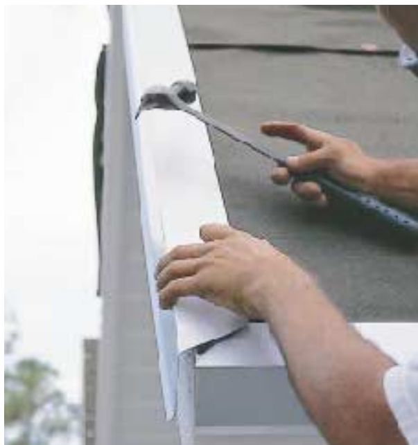
Figure 1. The same 3x3-inch flashing profile is used for the rake flashing and the drip-edge. The flashings are mitered at the corner.
