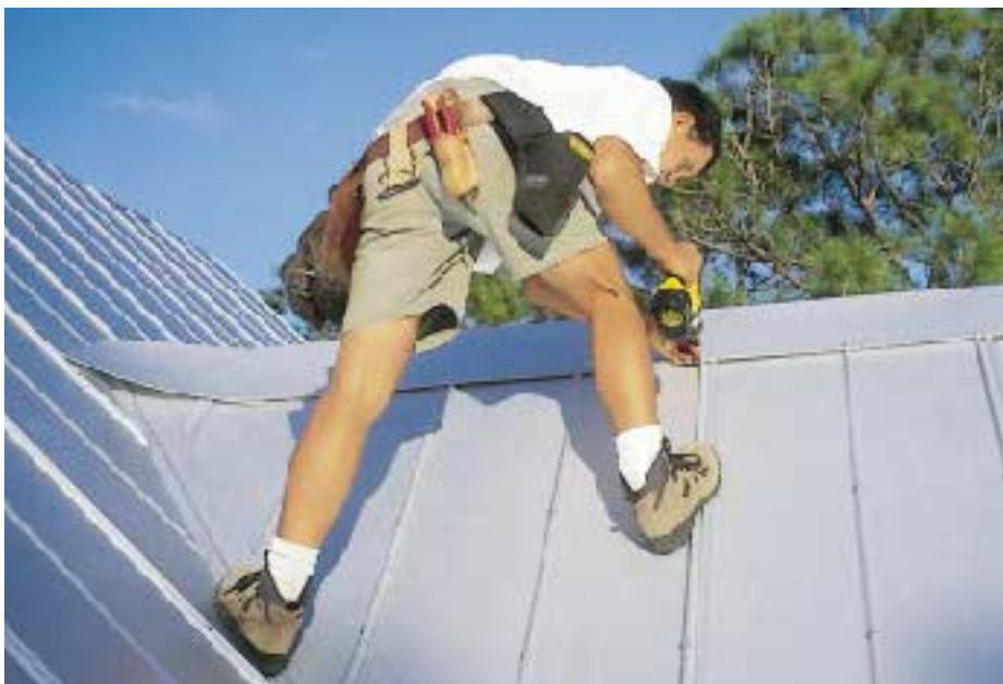
Figure 10. The last step is installing the 6x6-inch cap flashing.
