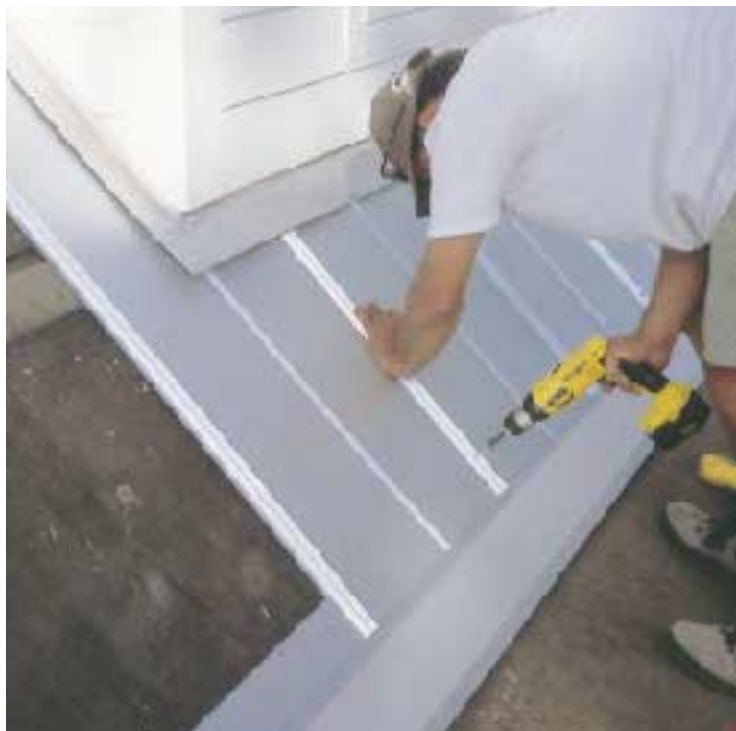
Figure 2. The L-flashing at wall intersections is installed before the siding goes up (left). This flashing is installed above the plane of the roof sheathing, to leave enough room for the roofing panels to be slid under it (right).
