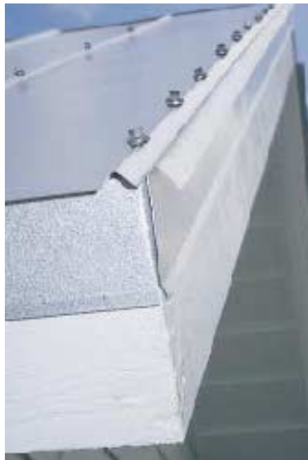
Figure 5. Roof panels are always installed square to the eaves. If you're lucky, and the roof is square, the panel will be parallel to the rake.
