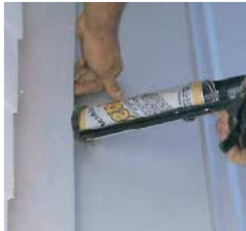
Figure 8. At wall intersections, it's important to install butyl tape or caulk between the L-flashing and the roof panels. Caulk can be omitted if one of the panel ribs falls under the flashing.
