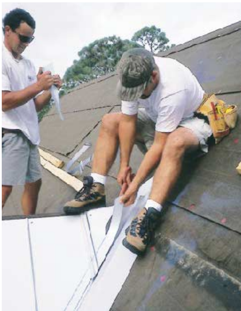
Figure 7. Where the panels meet a valley, the edges are trimmed to a chalk line after the panels are installed.
