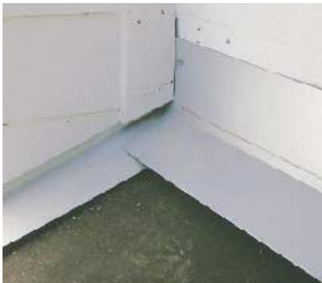
Figure 2. The L-flashing at wall intersections is installed before the siding goes up (left). This flashing is installed above the plane of the roof sheathing, to leave enough room for the roofing panels to be slid under it (right).
