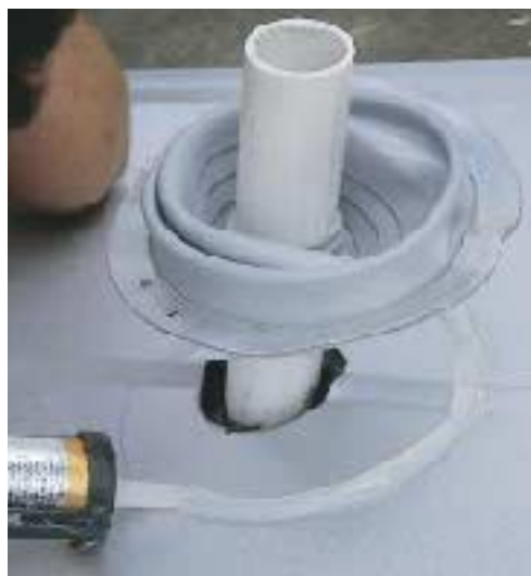
Figure 9. The best flashing for a plumbing vent is the Dektite boot. The boot is slipped over the pipe after the panel is installed. After installing a circle of caulk (left), the aluminum ring on the flashing is pressed down to conform to the ribs of the roofing panel. The flashing should be screwed every 3 inches (right).
