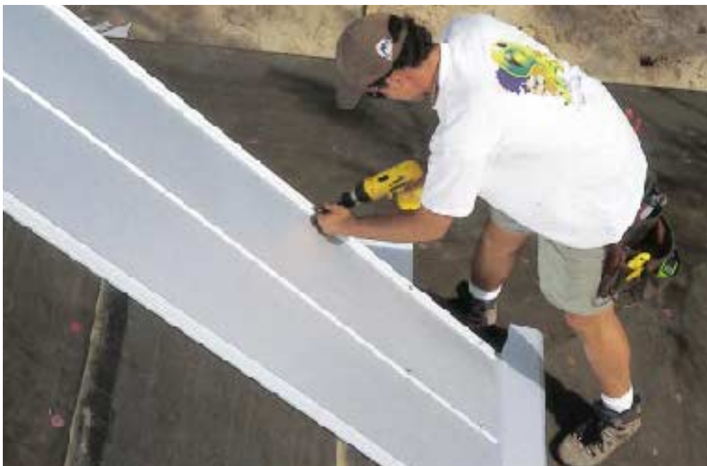
Figure 6. Fastening requirements vary, depending upon the panel configuration. Typical 5-vee panels are screwed every 16 inches along the ribs.
