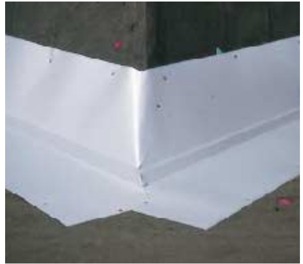
Figure 4. Where the tops of two valleys intersect a dormer ridge, one of the valleys is run past the intersection (left). Then the valley is carefully trimmed and folded to create a tight flashing (right). Use caulk at vulnerable corners.
