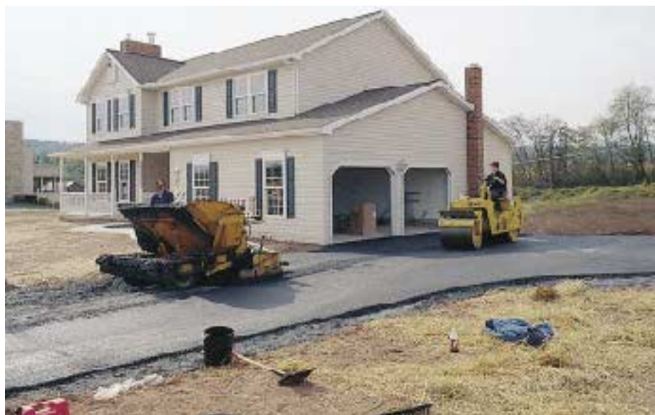
Figure 4. On an asphalt job, the PEX is protected with a layer of stone dust (foreground, top) before the hot asphalt is placed (center) and rolled (above).
