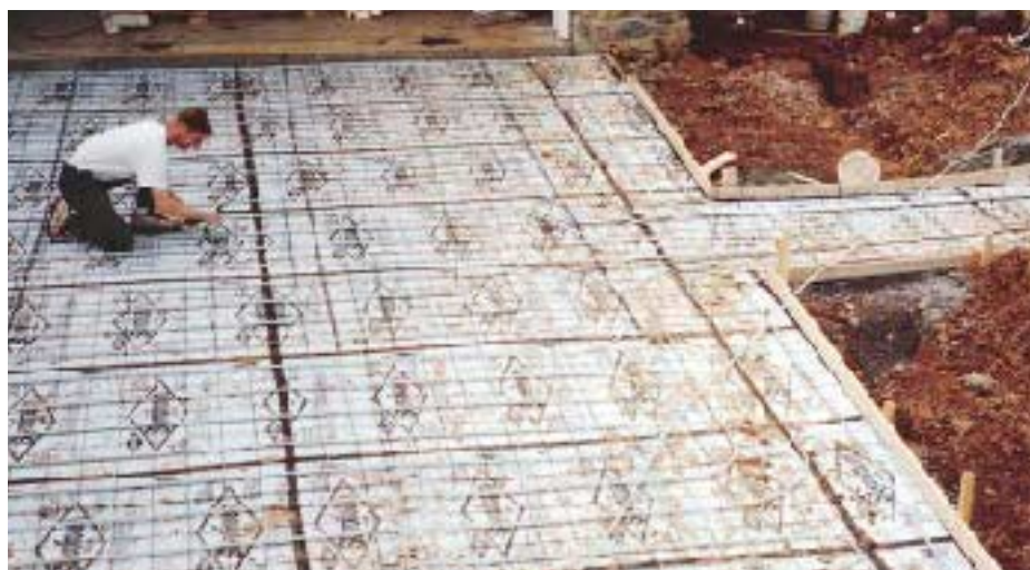
Figure 2. After the crushed stone base is spread and compacted, 1-inch extruded polystyrene board is laid over the entire snowmelt area (top). Next, sheets of wire mesh are laid out and the tubing is strapped to the grid (center). Finally, before the pour, the temperature and humidity sensor is positioned in a bed of mortar so that it ends up dead level with the final surface of the concrete (left) — a critical detail.
