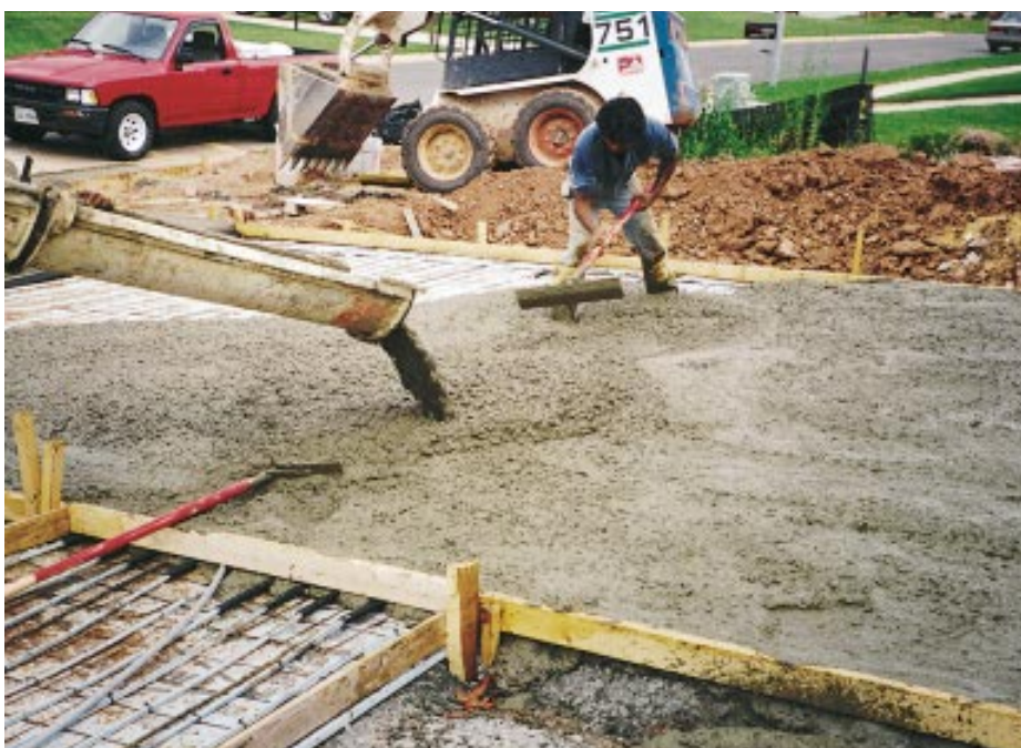
Figure 3. To avoid damage to the tubing, control joints should never be cut after the concrete sets. Instead, use plastic strips or a similar technique to form control joints when the concrete is placed. Sections of black closed-cell-foam pipe insulation protect the tubing against slight movement at control joints (top). The author recommends against lifting the mesh and tubing up into the concrete during the pour (above).
