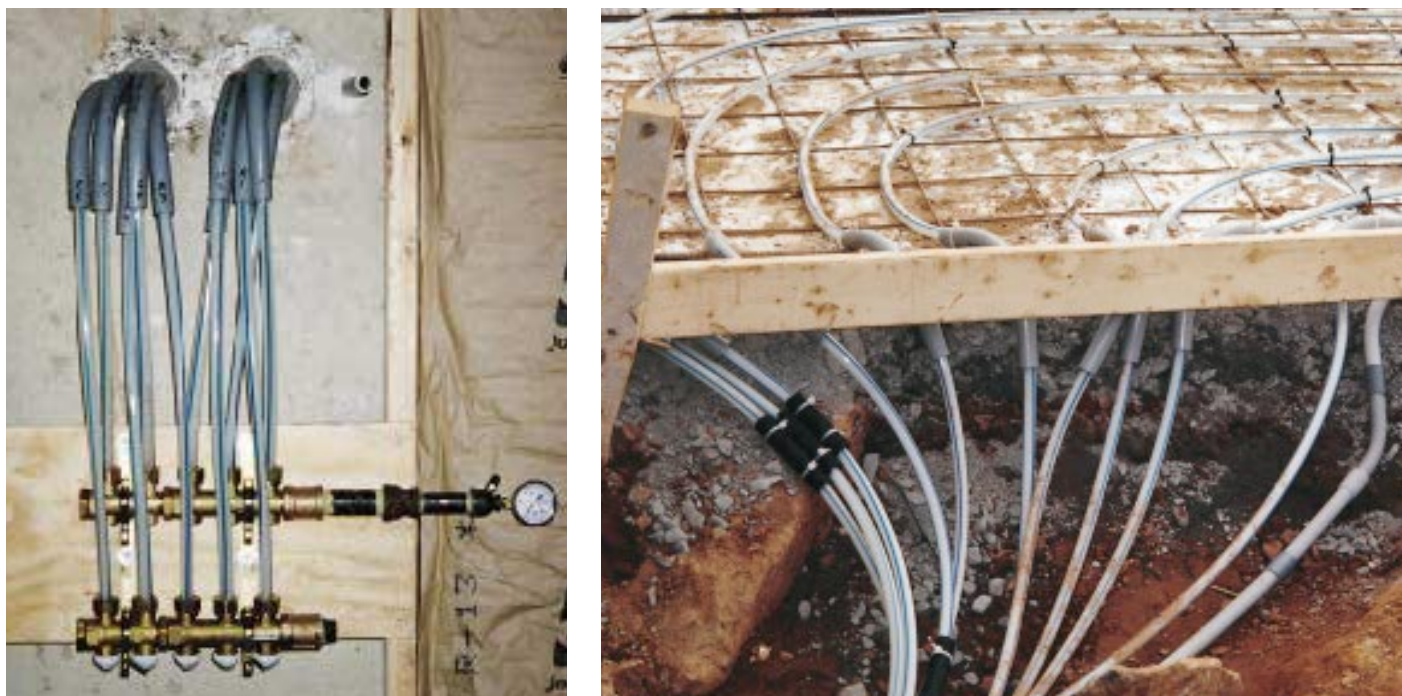
Figure 1. The piping for the snowmelt loops originates at a manifold in the basement or boiler room (left). Sleeves of PVC conduit protect the tubing where it passes through the foundation wall and up into the driveway slab (right). The conduit on the far right in the right-hand photo carries low-voltage wiring for the heat sensor embedded in the drive.
