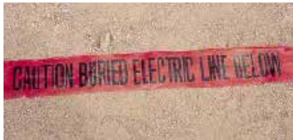
Figure 3. Locating color-coded marker tape 12 inches above the buried line is essential for safety.
