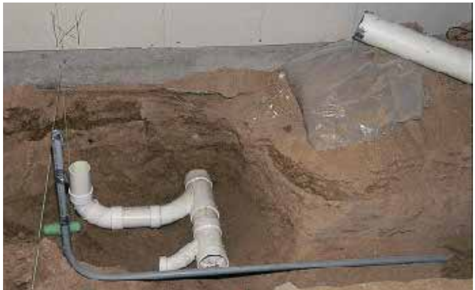
Figure 1. A stringline for reference helps everyone. On this job some walls were in place prior to pouring the slab, but the principles are the same.
