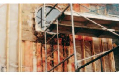
Water penetration has caused thousands of relatively new wood-framed buildings in British Columbia to rot. A government inquiry placed blame on faulty design, shoddy construction, and inadequate inspections.
