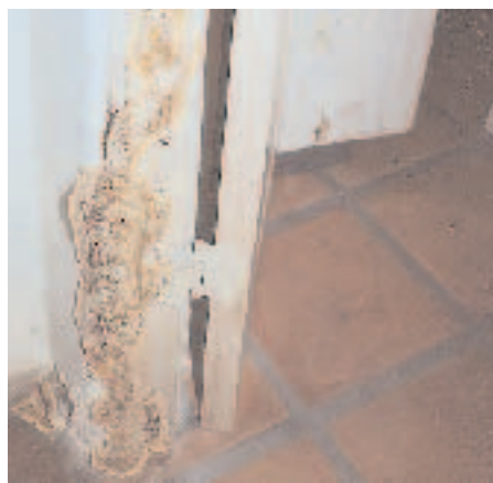
Unlike most wood-decay fungi, poria can attack wood in dry areas of a house, thanks to its ability to draw moisture from remote sources.
