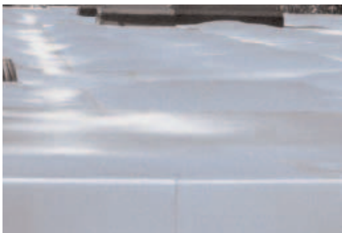
Some roofing contractors have reported problems with polyisocyanurate insulation boards shrinking or expanding after installation.
