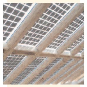
A model home in Burnaby, B.C., has a room with semi-transparent sloped glazing that includes photovoltaic cells laminated into the glass.
