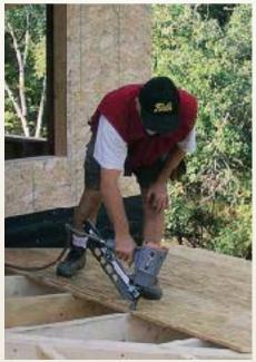
The author finds that gluing and nailing with ring-shank nails results in a problem-free installation.
