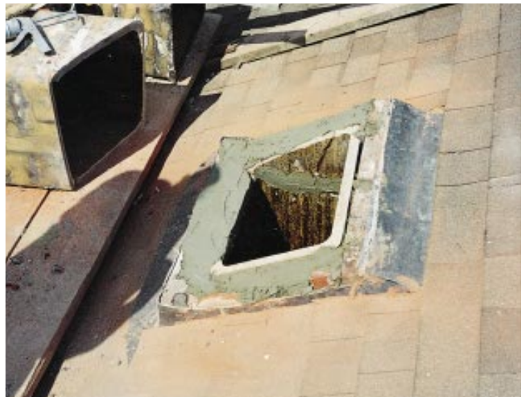
Figure 2. Using the roof to guide his circular saw, which is fitted with an abrasive diamond masonry blade, the author cuts through the lead and brick on either side of the chimney parallel to the slope (left). The flue tile is marked with a pencil, removed, cut, and replaced. Gaps in the brick are filled and parged with mortar to provide a smooth, even base for the lead pan (right). The basic layout is identical in new construction, minus finished roofing and flashing.
