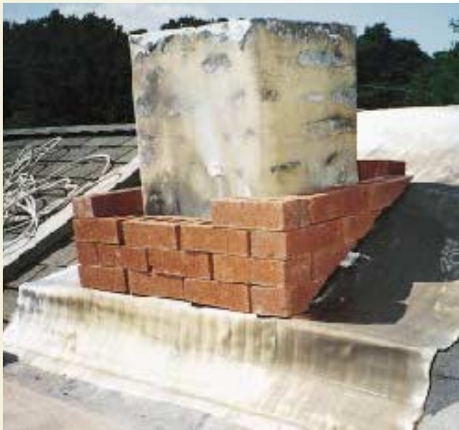
Figure 6. The author cuts and dry-lays all of the makeup brick courses on the pan, then sets them in mortar. Two vertical joints are kept mortar-free to serve as weepholes, allowing any penetrating water to drain from the pan.
