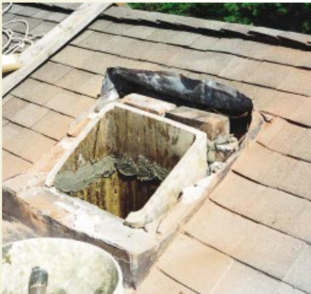
Figure 2. Using the roof to guide his circular saw, which is fitted with an abrasive diamond masonry blade, the author cuts through the lead and brick on either side of the chimney parallel to the slope (left). The flue tile is marked with a pencil, removed, cut, and replaced. Gaps in the brick are filled and parged with mortar to provide a smooth, even base for the lead pan (right). The basic layout is identical in new construction, minus finished roofing and flashing.
