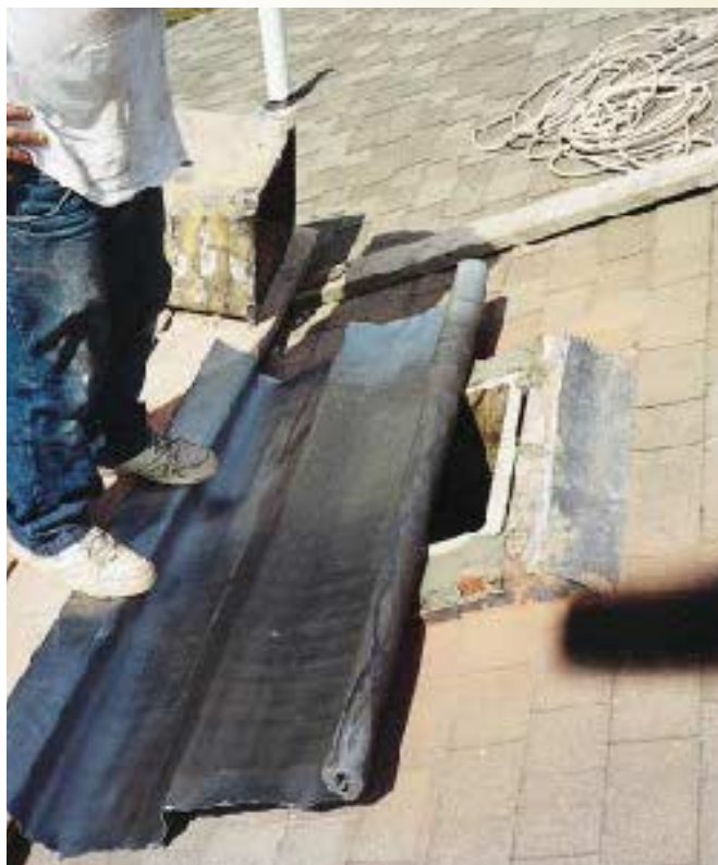
Figure 3. After the lead is cut to width while still rolled, it's laid out and centered over the chimney, leaving a 12-inch-wide skirt on three sides, with the excess run up the roof, at least three shingle courses high on a mid-roof chimney.
