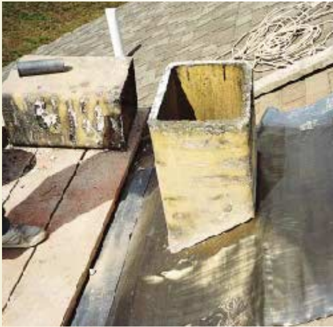
Figure 5. The remaining section of the cut flue tile is set in a heavy bead of joint repair mastic, surrounding the upturned lead berm. The mastic serves as an additional water stop, and helps to hold the flue in place on the lead during construction.
