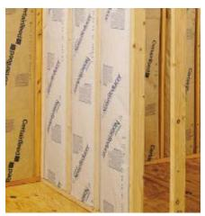
offer improved acoustical absorption when used to fill interior stud bays. The manufacturer claims the kraft-faced,  $3^{1/2}$ inch-thick batts add 4 to 12 points to the sound transmission class rating of the wall assembly. (Plan on using thermally-rated insula-
