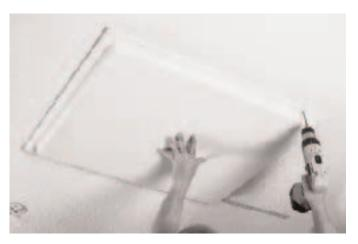
is made of paintable white ABS plastic, concealing a core of R-7 insulating EPS foam. Installation and removal are simple, with four special turnbuckle fasteners to hold the closed-cell gasketed mounting flange in place. Finished openings up to 23x30 inches can be covered for about \$50.
