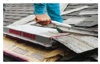
cuts on the new 18-inch-wide laminated shingles. The cutting table has an inlaid tape for quick reference. The shear costs \$233 including shipping and handling; replacement blades cost under \$20.
