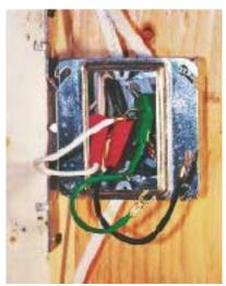
via a "pigtail" from a common wiring terminal. *Term-a-Nut Pigtail Connectors* make it simple, combining a twiston connector, flexible lead, and spade terminal in a one-piece wiring solution. The connector eliminates wire stripping and forming, and provides neat, uniform splicing inside the box. The connector is sold by
