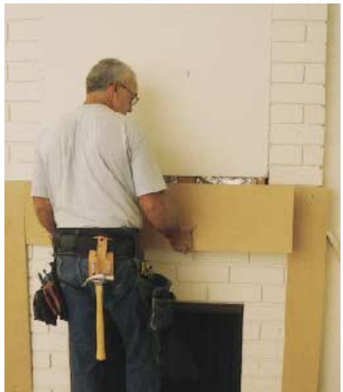
Figure 3. The pilasters must be dead parallel so that the frieze board fits snugly in between.
