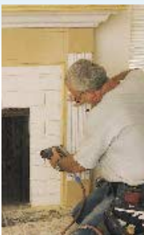
Figure 6. The frieze and end blocks get trimmed with crown.
