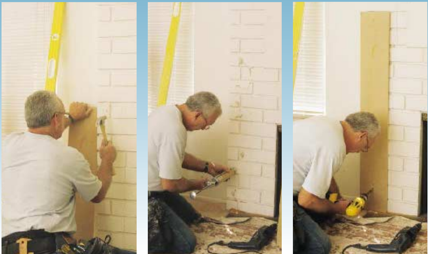
Figure 2. Masonry anchors (left) and construction adhesive (center) work together to secure the pilasters: The screws (right) hold the pilasters in place while the adhesive cures.
