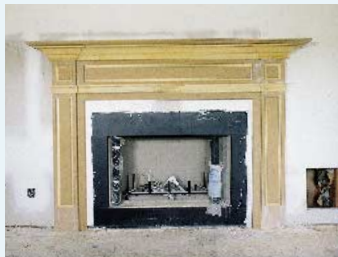
The completed buildout gets trimmed with panel molding and a collar molding to create an elegant painted mantelpiece.
