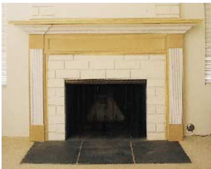
Figure 7. Panel molding around the inside of the surround (top left) covers up any cracks between the pilasters and the brick. The same panel molding dresses up the frieze (top right). A small molding around the top of the shelf completes the mantel, and it's ready for paint (above).
