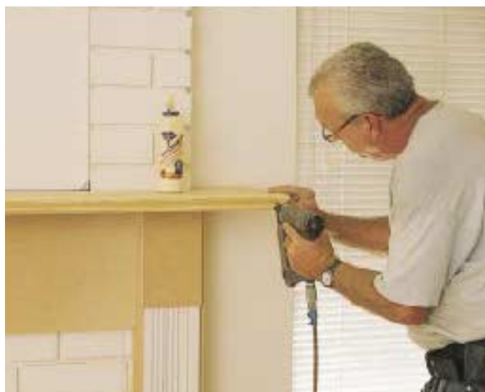
Figure 5. The mantelshelf consists of two pieces of \frac{3}{4} -inch MDF, scribed to the wall (top), nailed to the end blocks (middle), and trimmed with a nosing (above).
