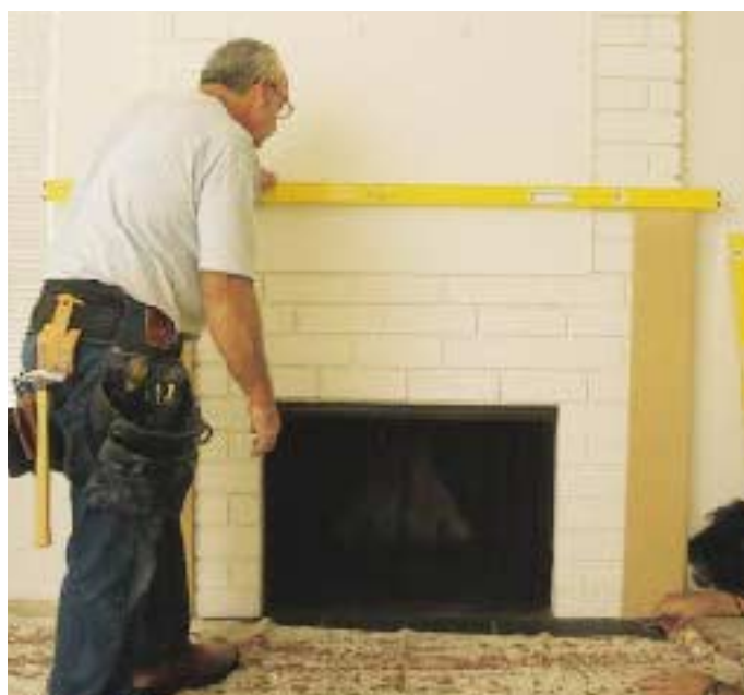
Figure 1. The mitered pilaster pieces are glued and pinned together (top), then scribed to the wall (middle). Before attaching the pilasters, the author makes sure the tops are level, scribing to the floor as needed (above).
