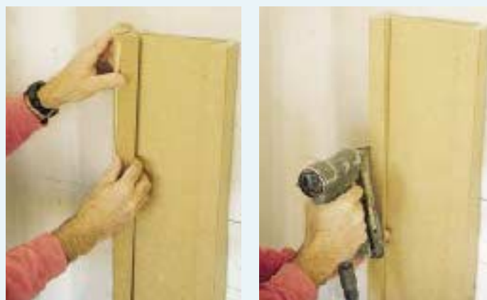
Strips of MDF mitered, glued (left), and pinned together on the pilaster base (right) provide a buildout for a paneled look.
