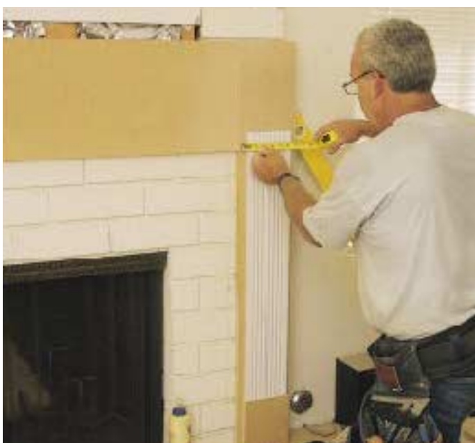
Figure 4. The base block installs with a \frac{3}{4} -inch reveal on both sides (top). The pilaster fluting (middle), which gets glued and nailed, gets a 1-inch reveal so that it steps in slightly from the base block (above).
