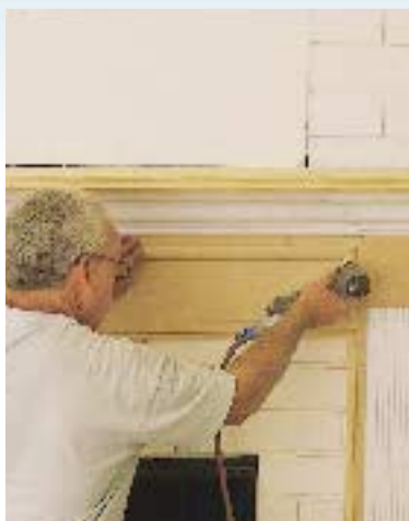
Figure 6. The frieze and end blocks get trimmed with crown.
