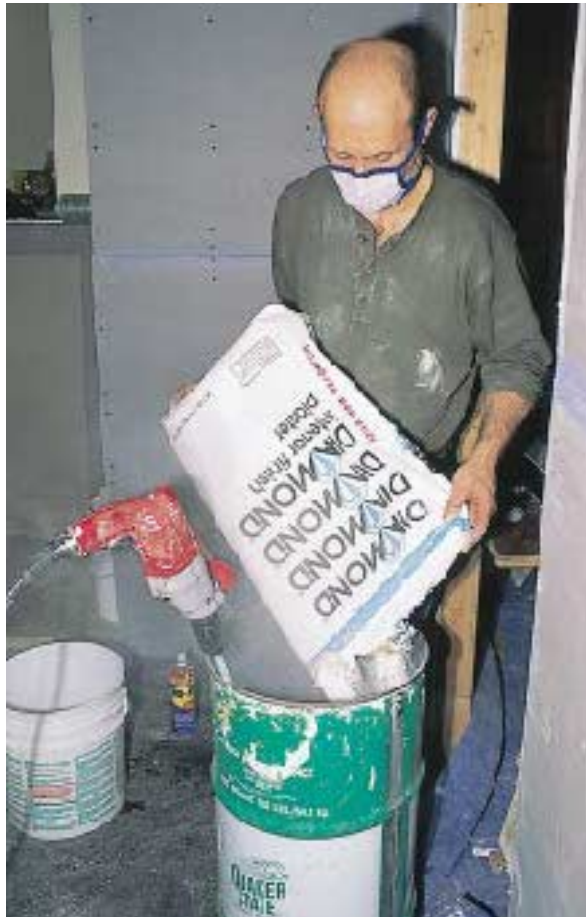
Figure 3. Plaster is highly alkaline, so it’s a good idea to wear dust protection during mixing, the dustiest part of the job. Use cool, clean water for a predictable mix, avoiding temperature extremes, which affect setting time. A recycled lube container controls the splatter of a two-bag mixing operation.
