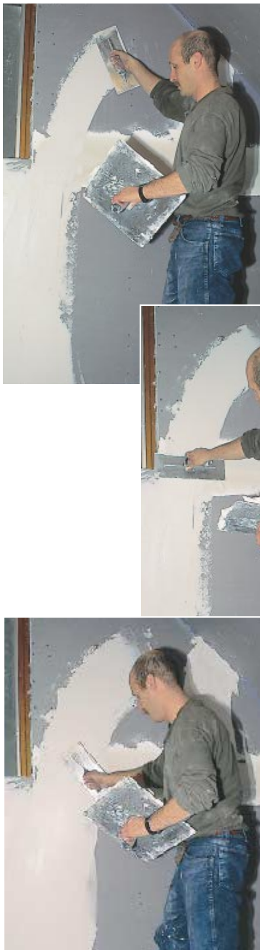
Figure 4. After scratching the panel seams, the author applies plaster in arcs, sweeping up to spread, down to embed, and back up to erase the trowel mark. The trowel never leaves the surface during application.
