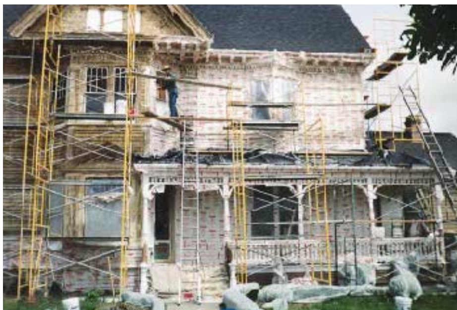
Figure 4. During stripping and repainting operations, it's a good idea to protect shrubs from chemical splatter with a landscape fabric.
