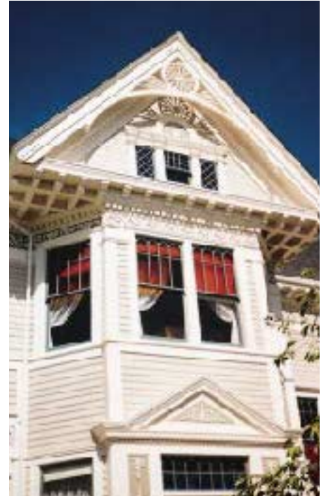
Figure 7. After neutralizing the stripped surface with an acid solution, the author allowed the wood to dry for more than two months before repainting with two coats of primer and two topcoats.
