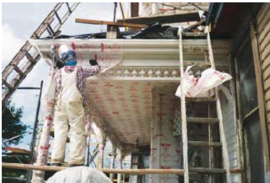
Figure 5. The paper is carefully pressed into place in an effort to eliminate air bubbles, which would prematurely dry the stripper.
