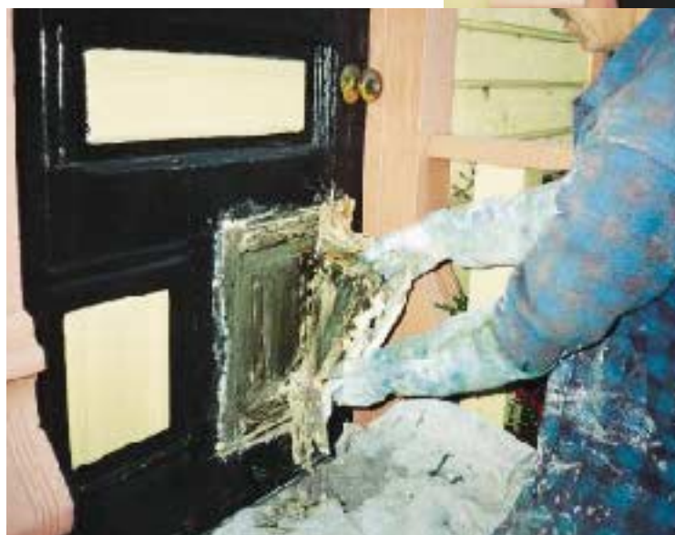
Figure 3. Before starting in on the entire house, the author tested a small sample area to determine how thick to apply the stripper, and how long to leave the paper in place.
