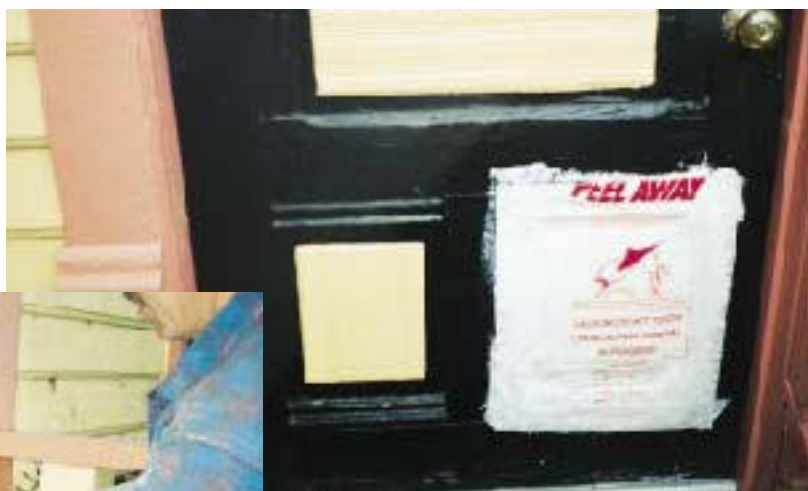
Figure 3. Before starting in on the entire house, the author tested a small sample area to determine how thick to apply the stripper, and how long to leave the paper in place.
