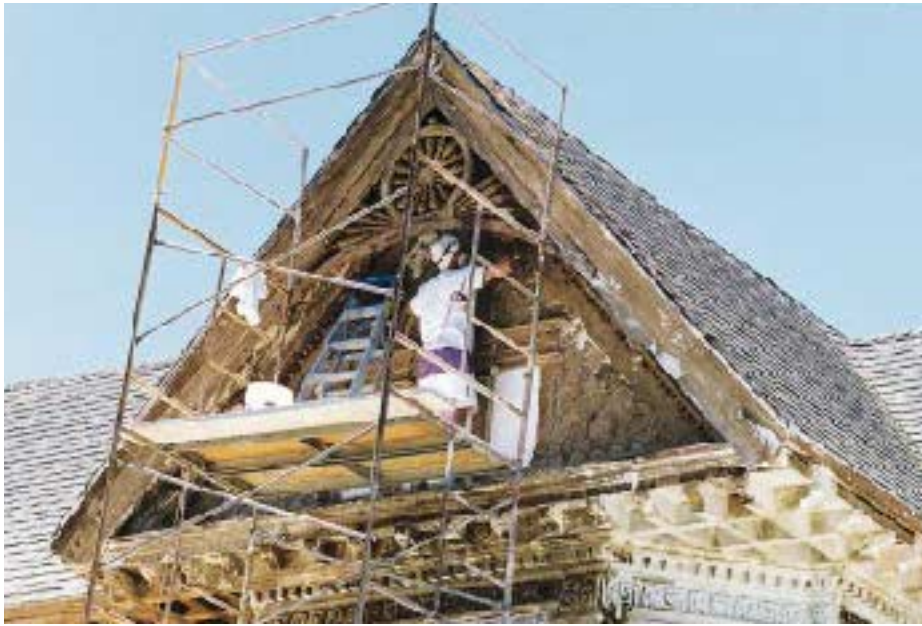
Figure 6. After stripping, the remnants of the original painted surface are removed with small picks and scrapers, a hose and scrub brush, or by pressure-washing.
