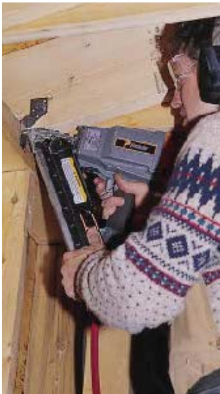
Figure 3. The brass-coated titanium probe at the tip of the Paslode Positive Placement nailer makes it easy to locate the nail holes in metal hangers. The probe pivots out of the way as the nail is driven.
