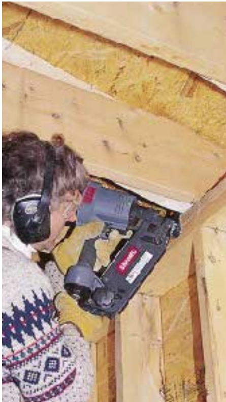
Figure 4. When using the Senco nailer, it's important not to push the gun forward or else the nail will not fire straight.
