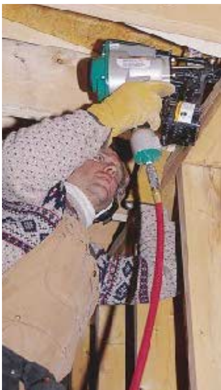
Figure 2. The Max CN601J coil nailer holds 100 hanger nails at a time. The location of the safety release arm alongside the nail (left) makes it tricky to see and place the nail when working lefthanded.
