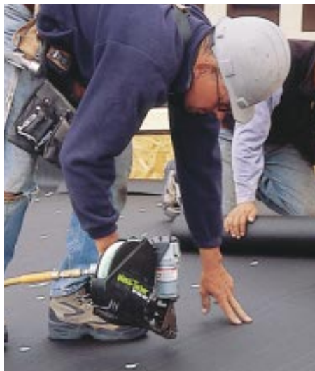
Figure 1. The Plasti-Tacker Pro makes fast work of 1 1 / 4 - to 2-inch nails with plastic caps.
