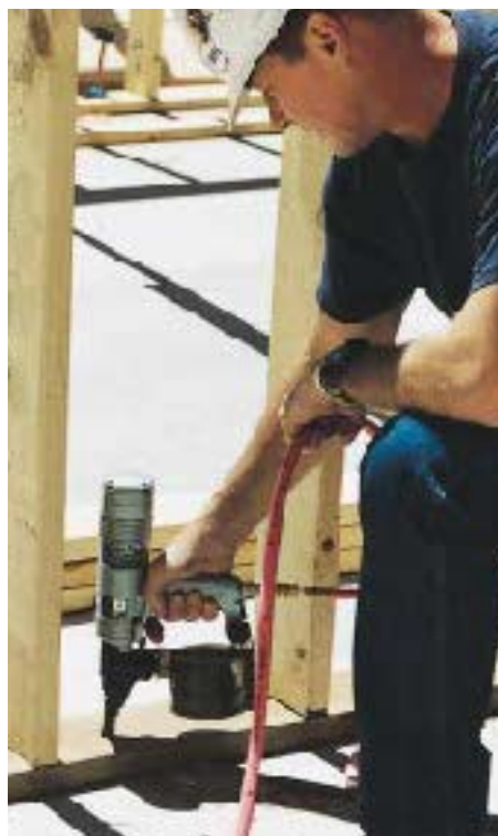
The Hitachi NC65AC nailer in action.
