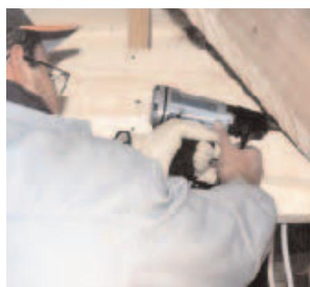
Compact size makes the AG125 ideal for nailing in tight places (above). It even worked well when used to drive spiral round-top nails through metal lathe, foam, and adobe (right). The Decade Vibration Reducing Gloves come from Chase Ergonomics (P.O. Box 92497, Albuquerque, NM 87199; 800/621-5436; [www.chaseergo.com](http://www.chaseergo.com)).
