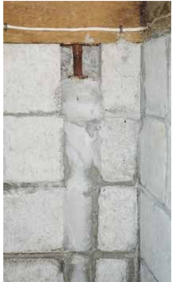
Figure 4. Temporary steel columns are grouted into place as part of the permanent foundation. Gaps in the blockwork provide access and ventilation.
