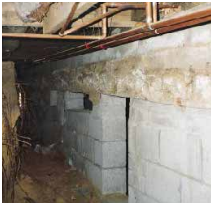
Figure 5. Old meets new at the basement stair landing, on the way down to the full-height cellar (above left) of this addition. On the other side of the wall is the original crawlspace (above right). The excavated area has been backfilled by hand to the top of the poured half-wall. The finished addition sits behind the original house (left).
