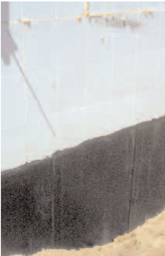
Figure 4. Membrane overlaps are pressure-bonded using a hand roller, then treated from bottom to top with proprietary sealant. Horizontal membrane terminations are caulked with mastic to complete the barrier system.
