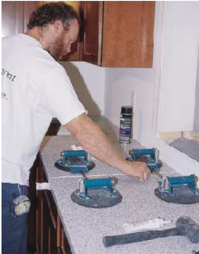
Figure 8. Turnbuckles attached to power grips (the suction-cup tools used for moving glass) can be used to draw together a solid-surface joint. This clamping system is especially convenient for field seams, where bar clamps can be awkward.
