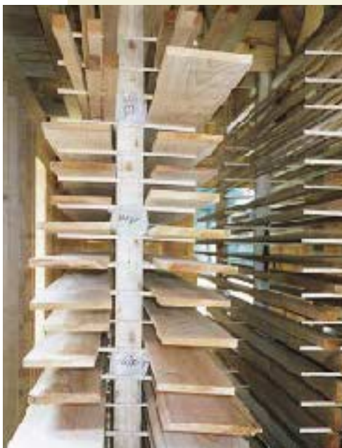
A site-built drying rack is a necessity for prefinishing on the job.
